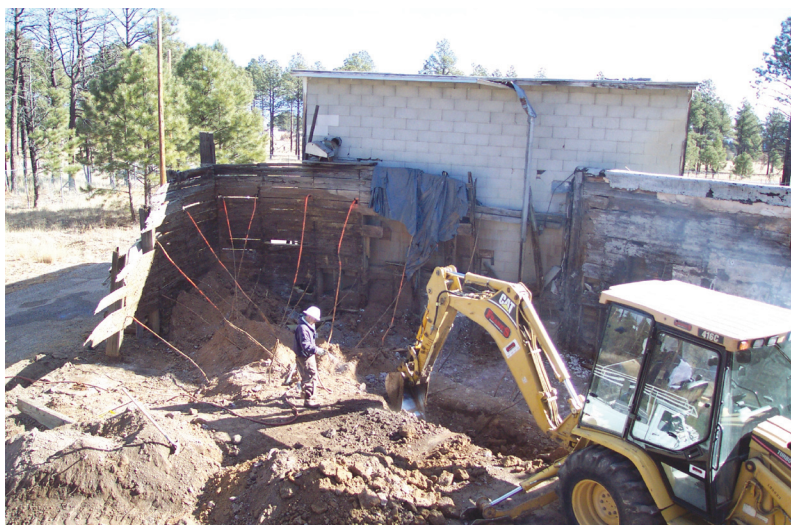
Phase 1 reconstruction of the earthen berm and berm retaining wall.
