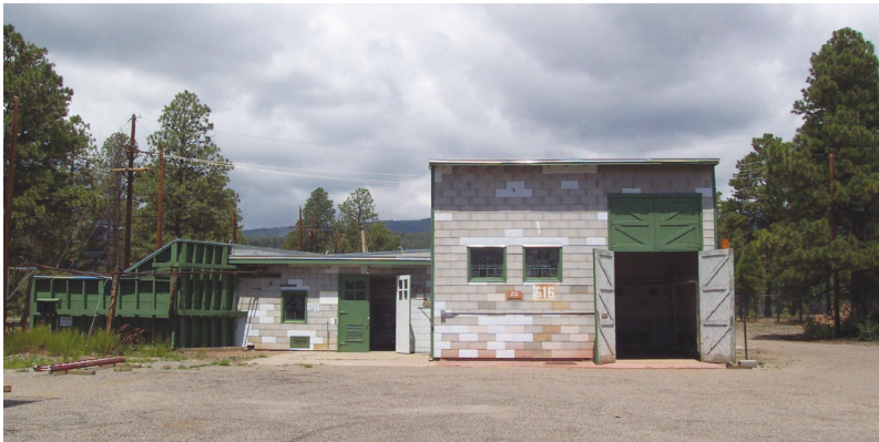
Buildings 516 and 517 at V-Site restored to their original 1944 condition.
