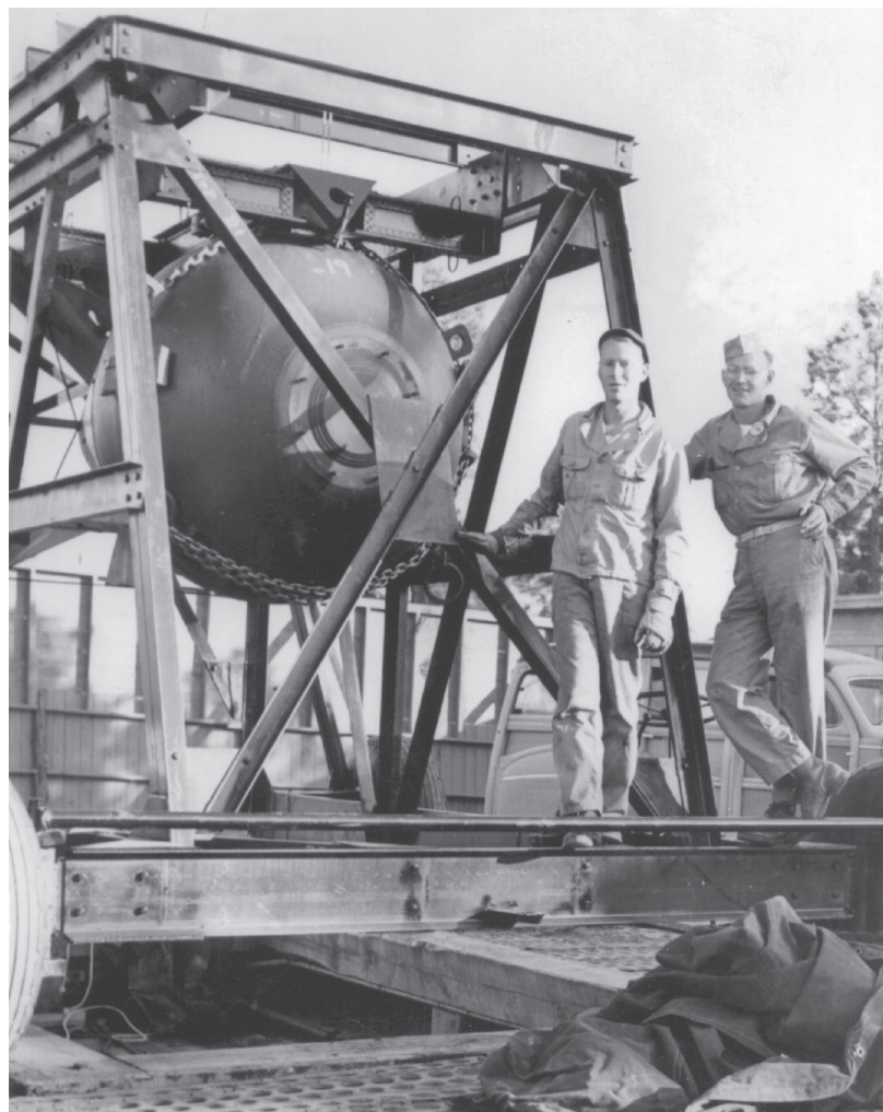
Fat Man assembly at V-Site.
