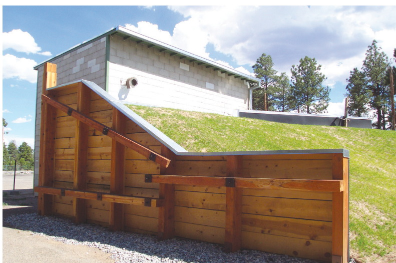
Reconstructed earthen berm and retaining wall.
