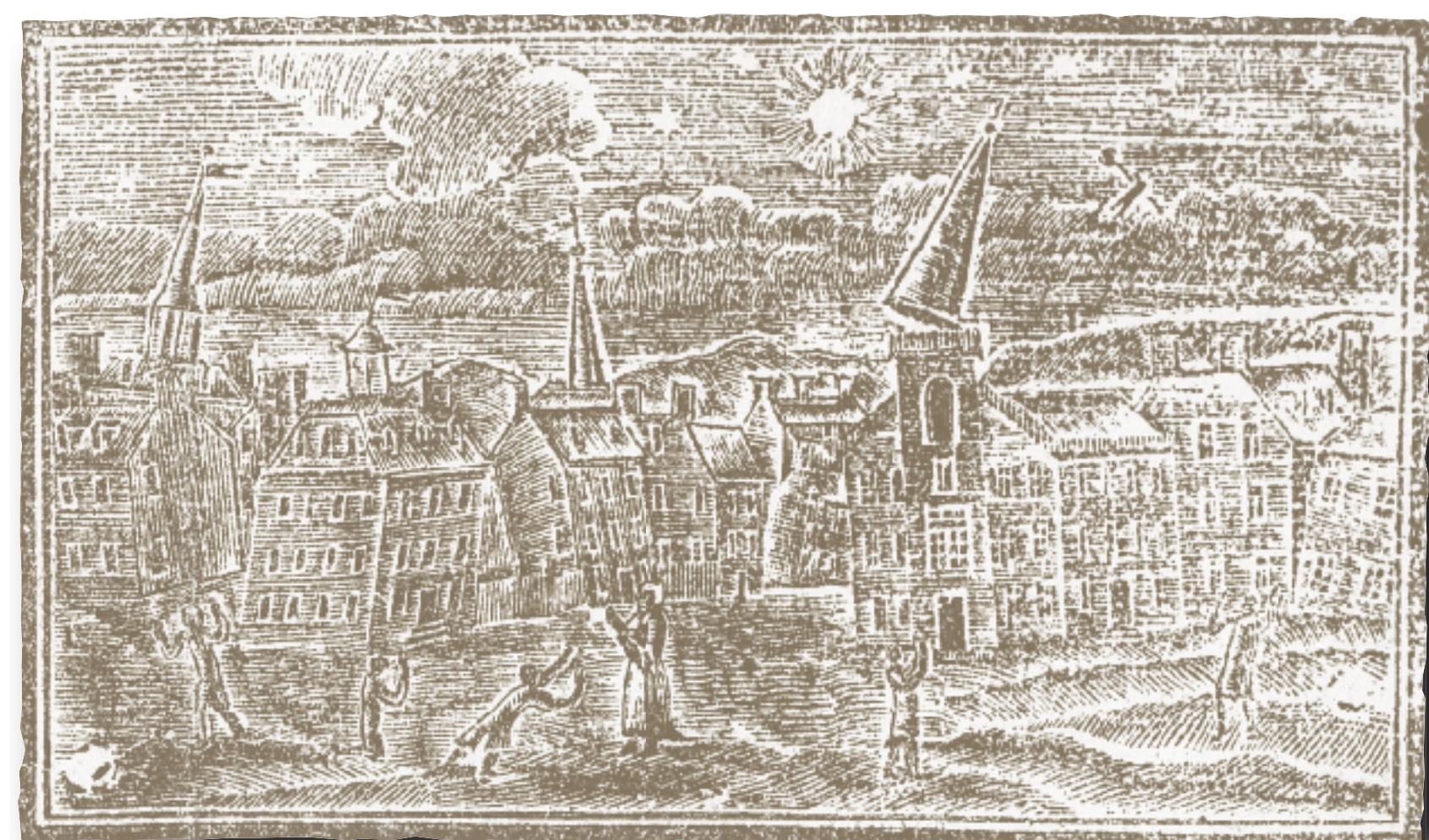
Old woodcut illustration showing contemporary account of damage to Boston, Massachusetts, during the Cape Ann earthquake of November 16, 1755. Shaking was strongest northeast of Boston. The magnitude 6.0 quake caused considerable damage in Boston, knocking down or damaging as many as 1,800 chimneys and collapsing brick walls of several buildings. (Reproduction of woodcut courtesy of the Trustees of the Boston Public Library.)
