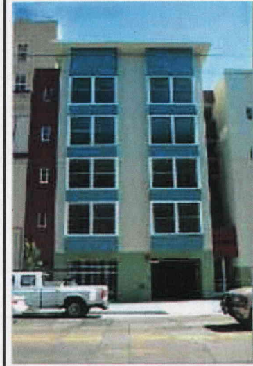
CERF helped develop Habitat for Humanity's new eight-unit apartment building in downtown San Francisco.
