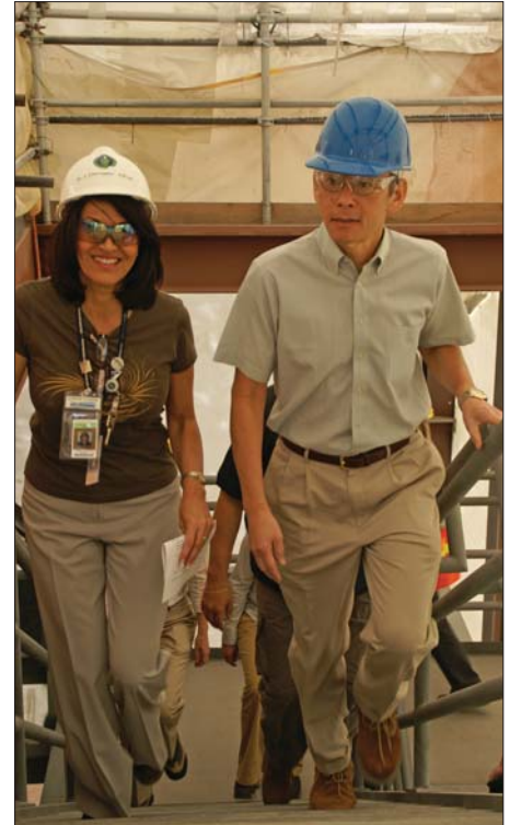
Shirley Olinger, Manager of DOE's Office of River Protection at Hanford and Secretary Chu climbed over 100 steps to reach the current top elevation of Hanford's Waste Treatment Plant Pretreatment Facility. When complete the facility will be twice as tall.
