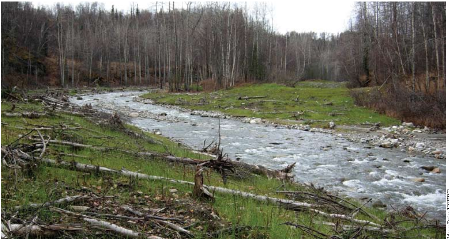
Woody debris and grasses planted on the banks held this restored bank in place during hard floods.
