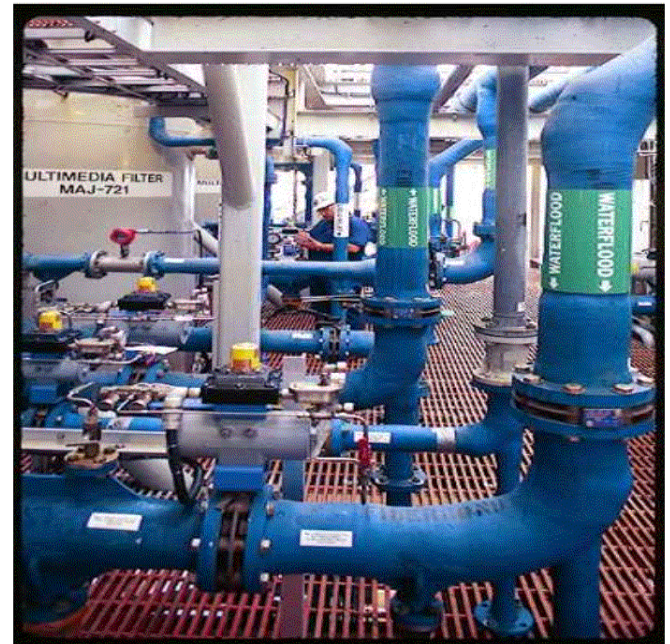
An example of Specialty Plastics' joining and fitting of composite-to-composite and composite-to-alloy pipe segments.
