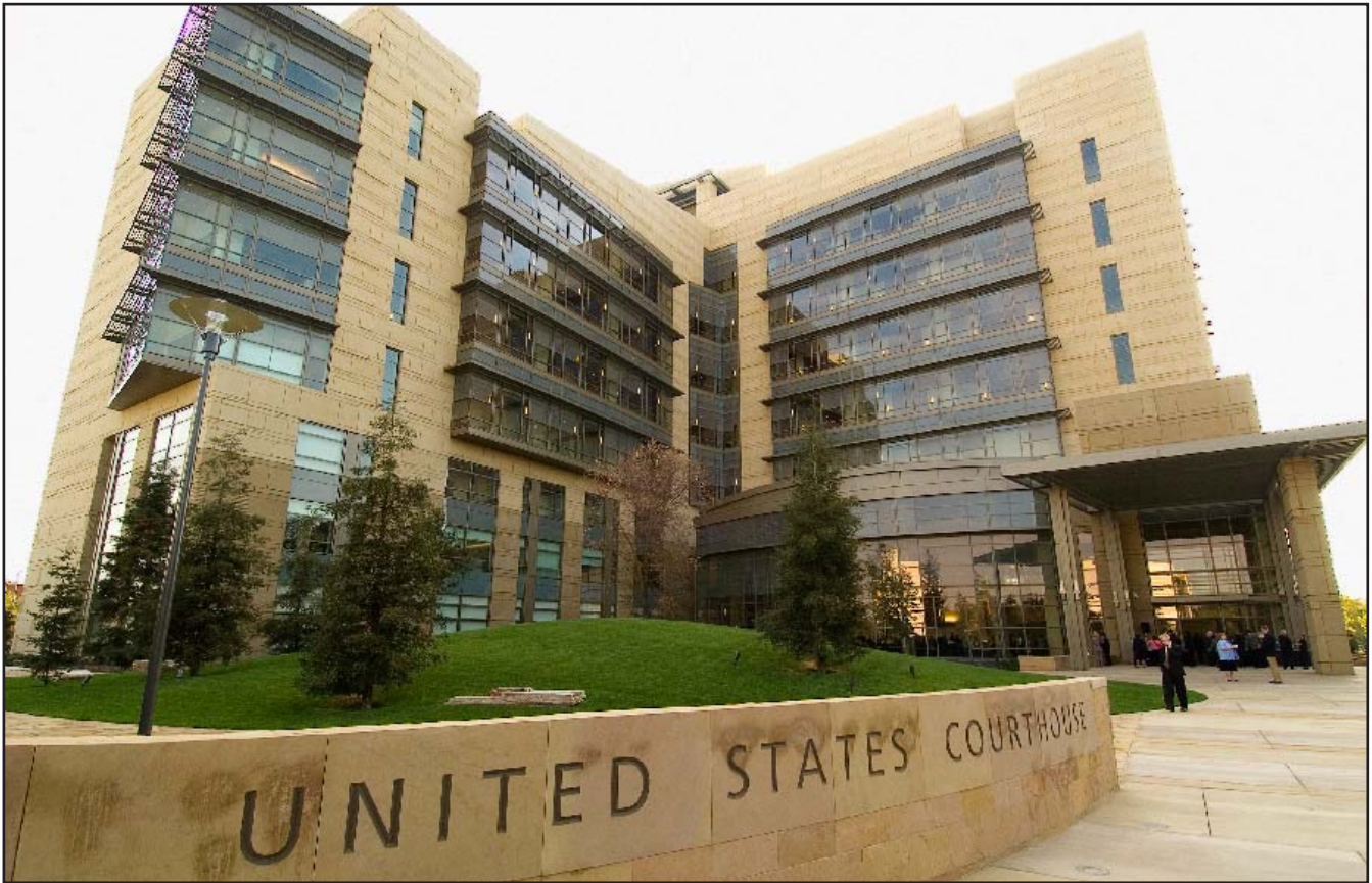
The new U.S. courthouse stands nine-stories tall at Tulare and O streets in downtown Fresno.
