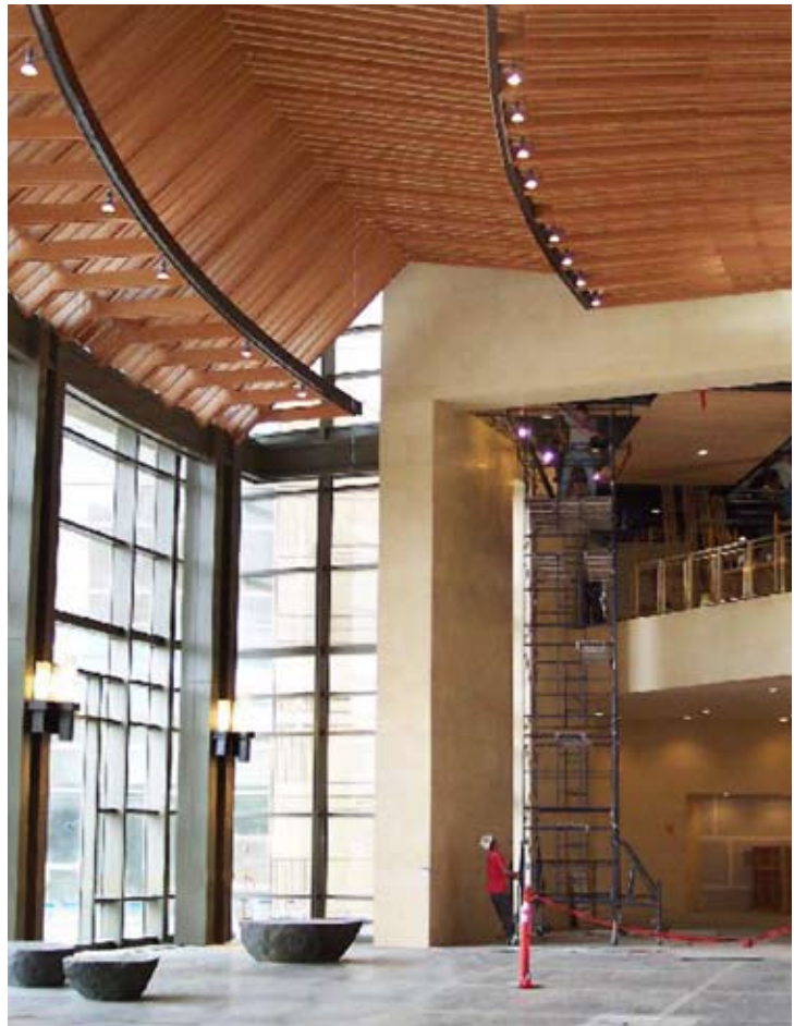
Workers move scaffolding in the lobby of the new Fresno courthouse.
