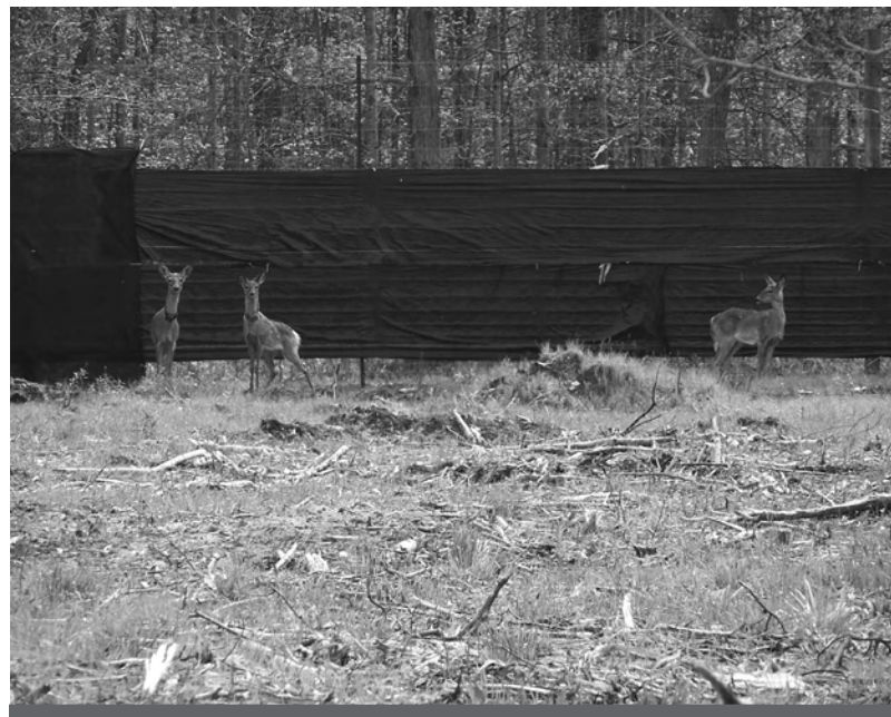
CWD Barrier Fence. (Photo by: Kurt VerCauteren)
