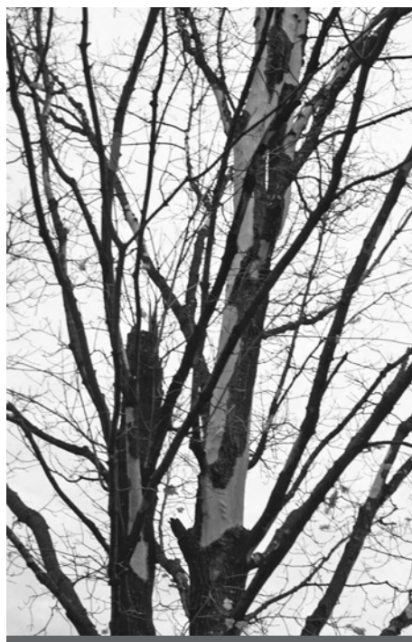
Tree damage by squirrels. (Photo by: USDA Forest Service, North Central Research Station)
