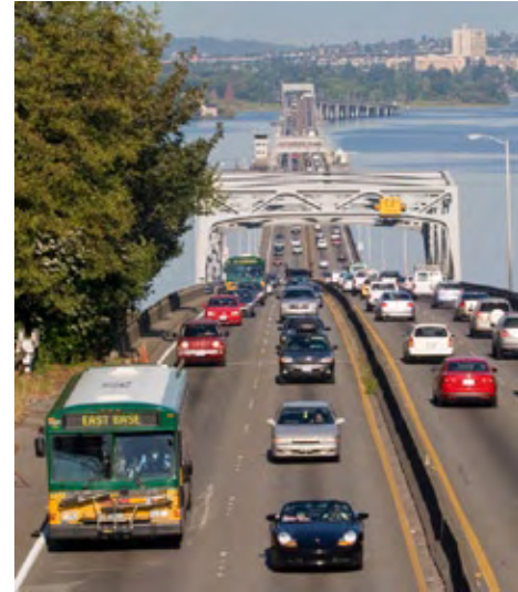
KCDOT is involved in plans to replace the Evergreen Point Bridge.
