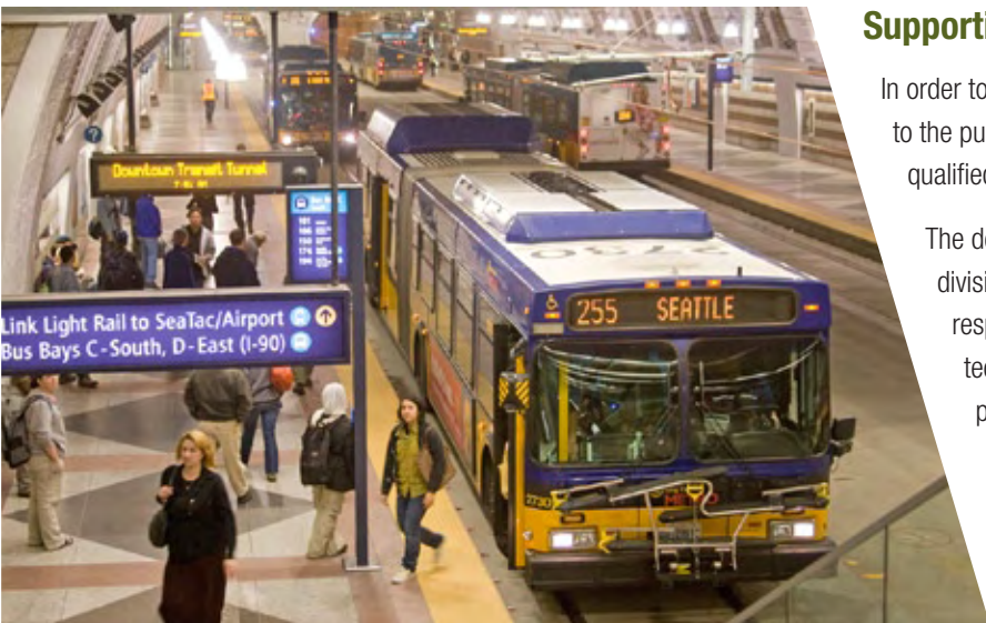
The retrofitted Downtown Seattle Transit Tunnel reopened in September 2007
