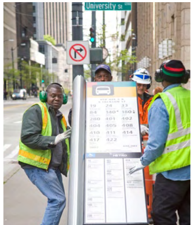
Transit crews install a prototype of a new bus stop sign.
