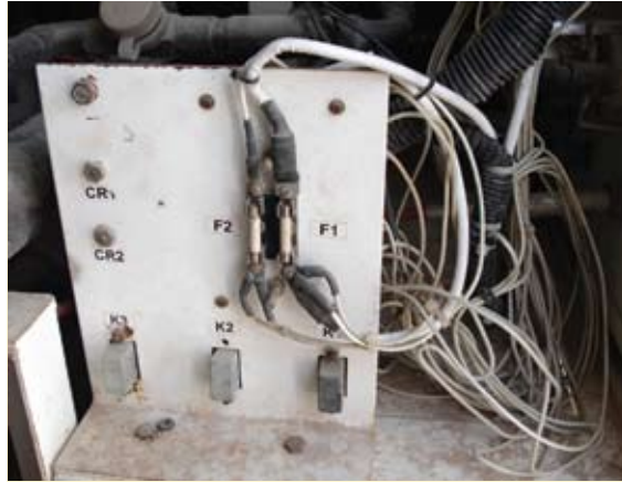
Proper fuse layout
