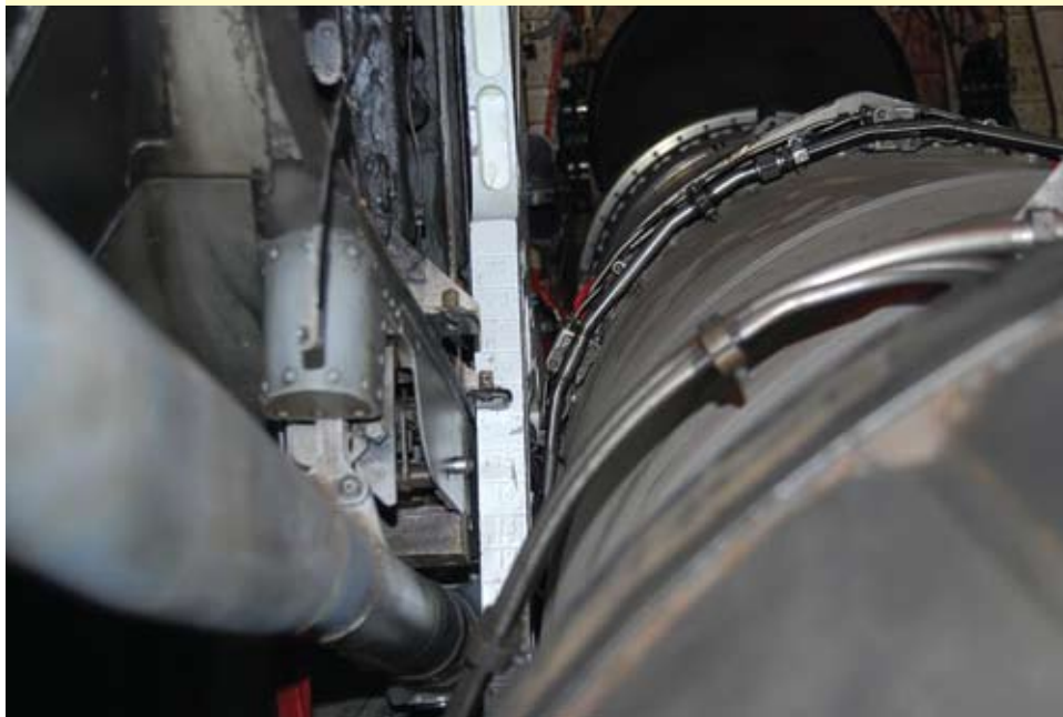
Engine shift inboard area between tailhook and engine is where the author had been standing (below).
