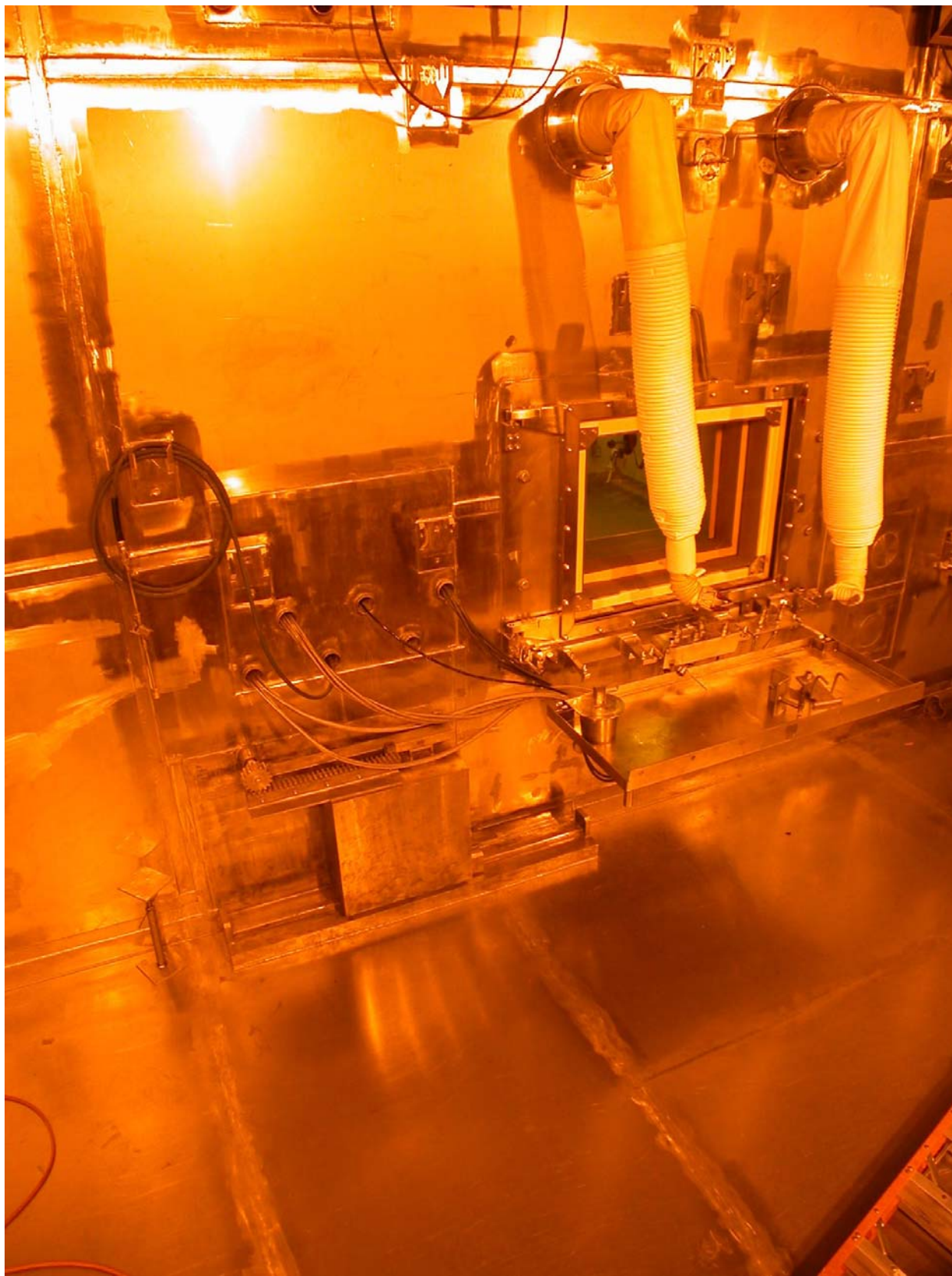
Fig 5.2-66. Input enclosure near workstation 3.
