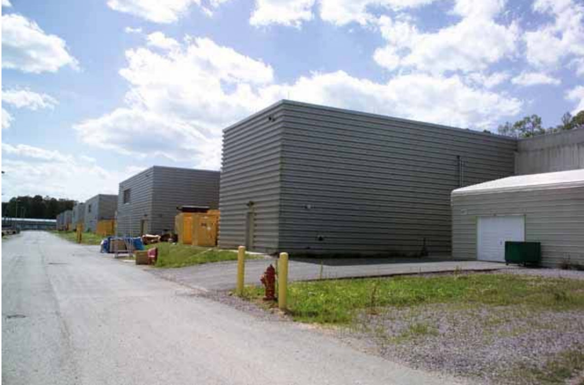
Fig. 5.5-5. Westward view of the Klystron Building.
