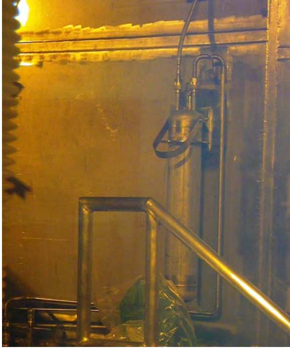
Fig. 5.2-81. Gold adsorber in service bay.
