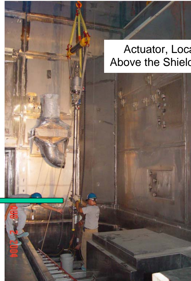
Installation of the valve
