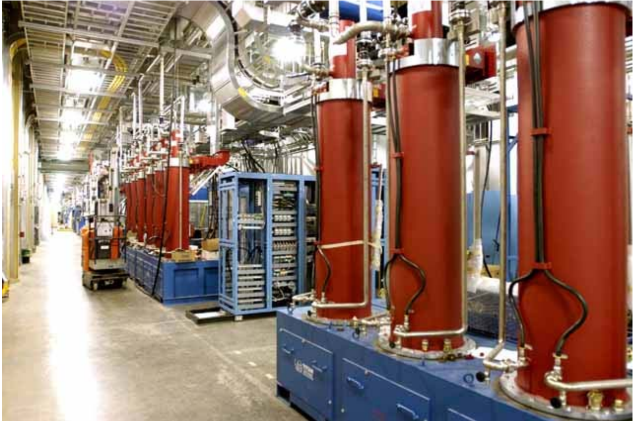
Fig. 5.1-18. Snapshot of the klystron gallery with some of the 81 klystrons feeding the superconducting linac.
