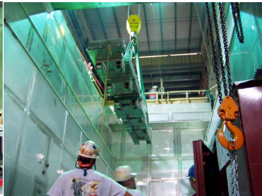
Being lowered into service bay
