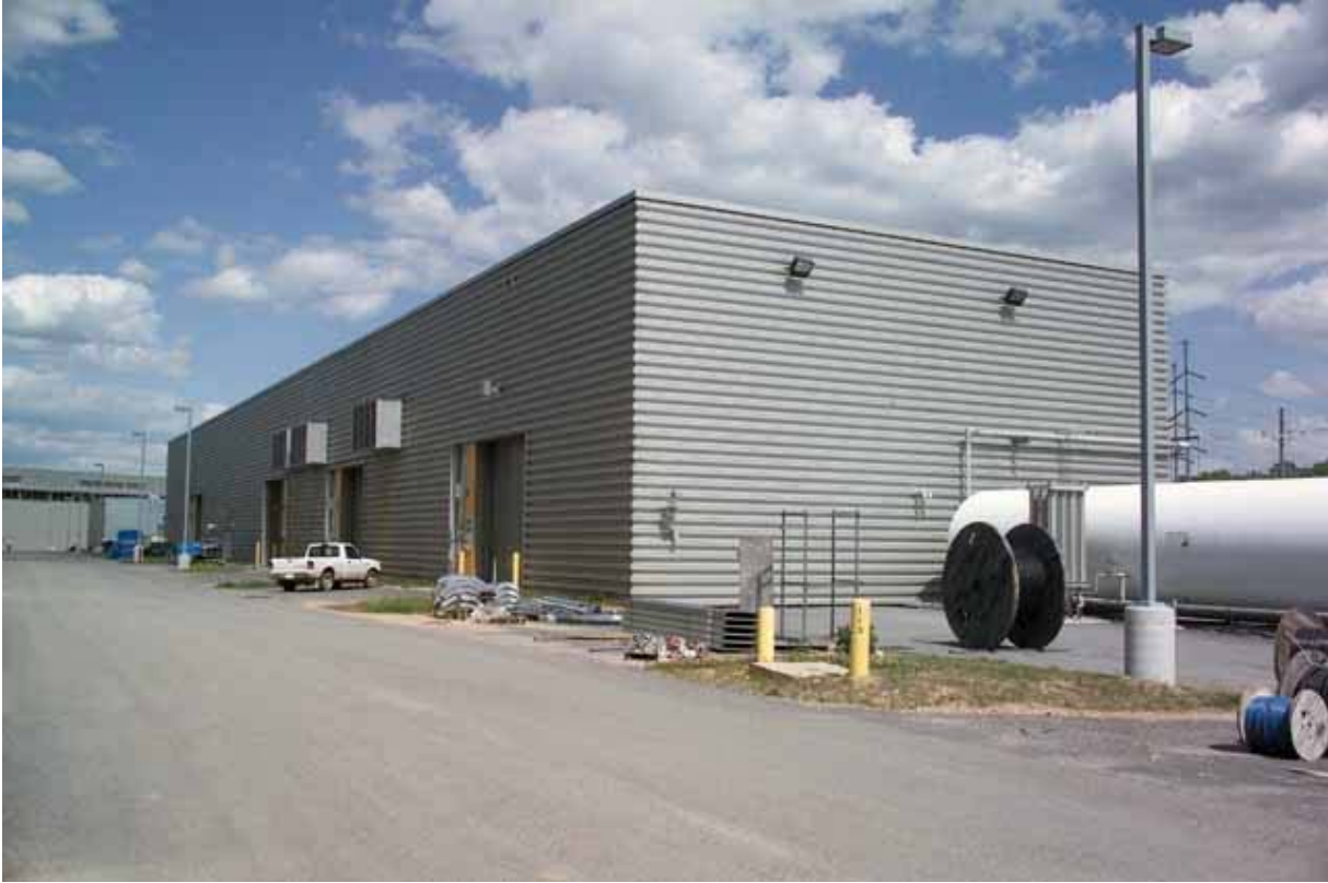
Fig. 5.5-6. Eastward view of the CHL Building.
