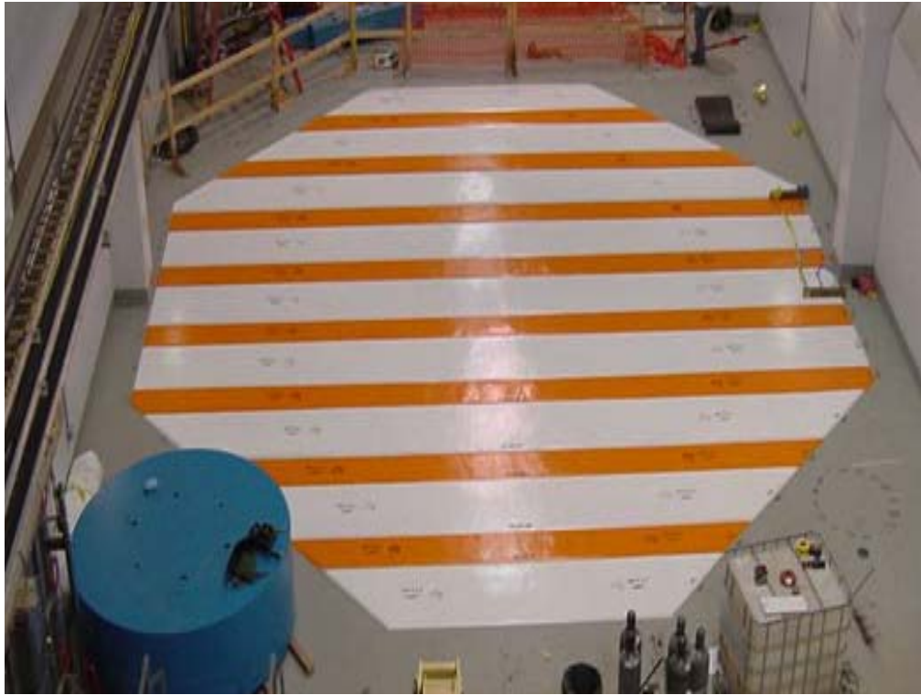
Fig. 5.2-53. Shine shield “T” beams installed.
