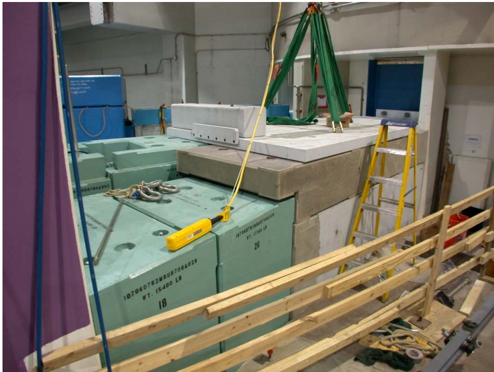
Fig. 5.3-15. Final shielding being installed on Magnetism Reflectometer and Liquids Reflectometer incident beam line.
