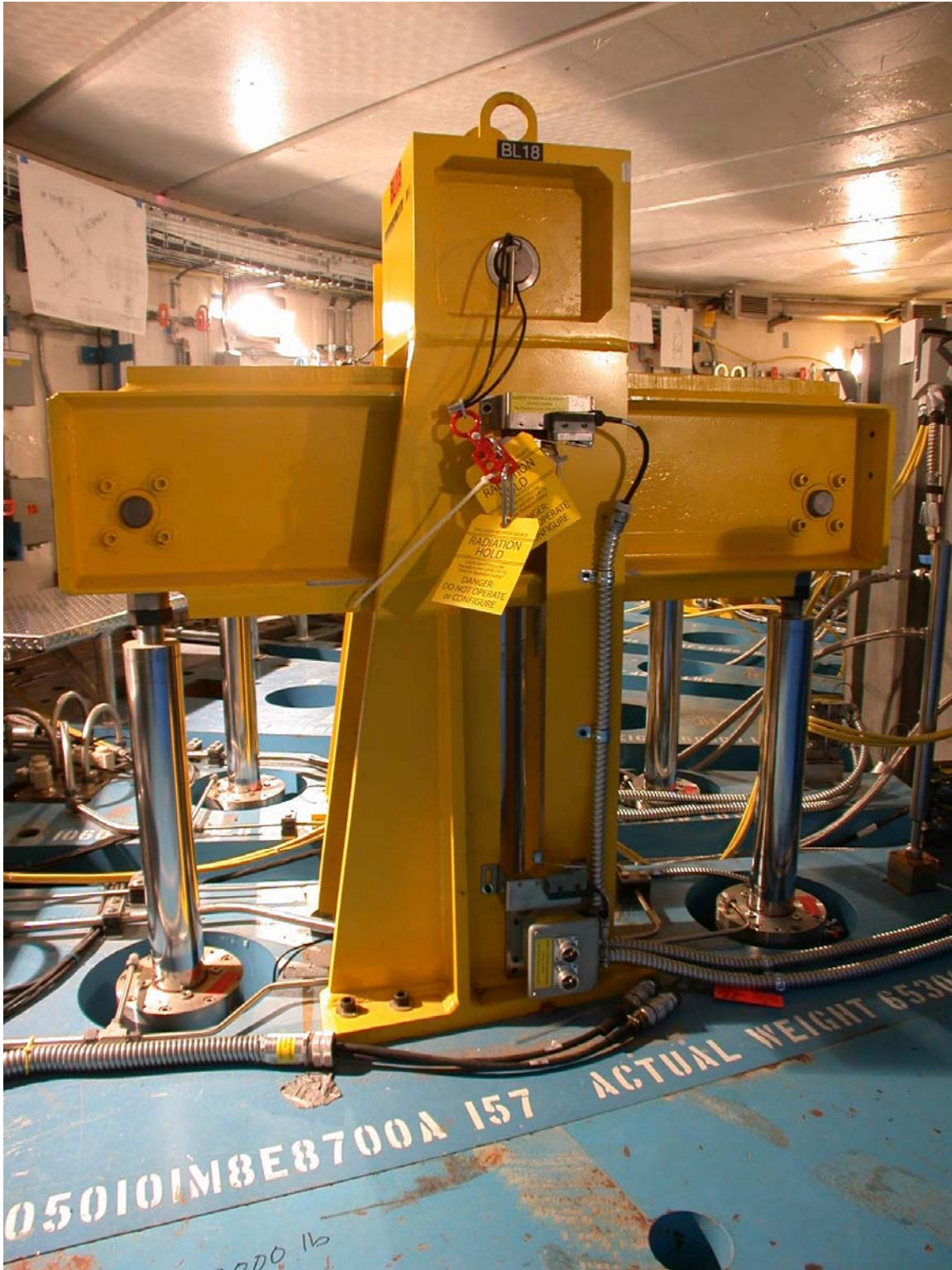
Fig. 5.2-50. Typical shutter drive system on top block.
