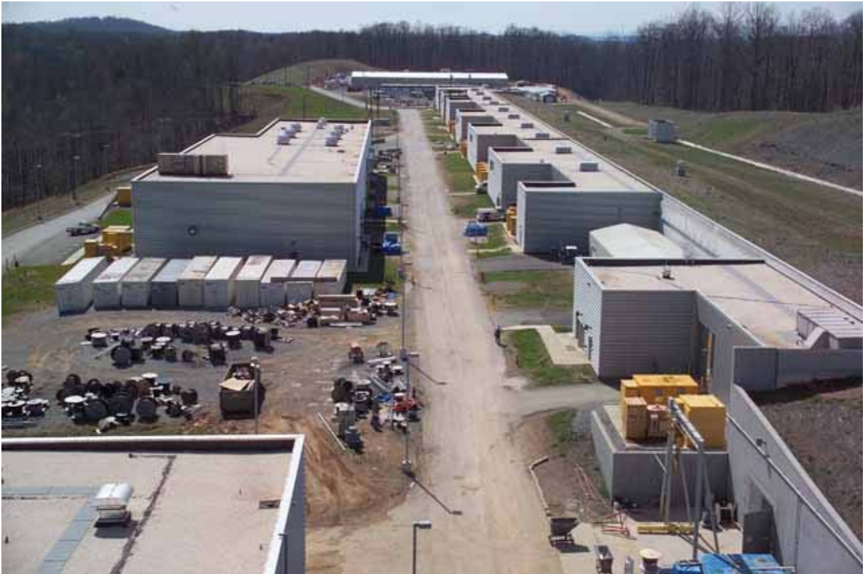
Fig. 5.5-4. Aerial view of the RF Building (left), the Klystron Service Building, and Klystron Building (right).
