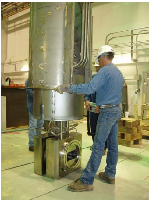
Fig. 5.2-29. Lower proton beam window assembly before and after installation.
