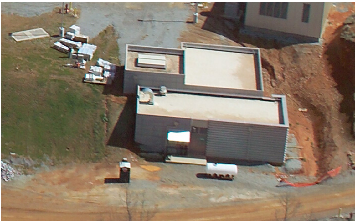
Fig. 5.5-20. Aerial view of the ring injection beam dump.
