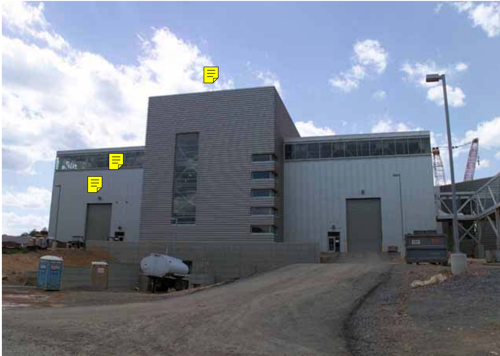
Fig. 5.5-19. Northward view of the completed Target Building.
