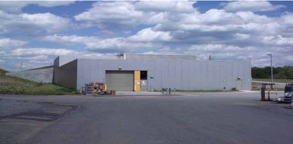
Fig. 5.5-2. Eastward view of the Front-End Building.
