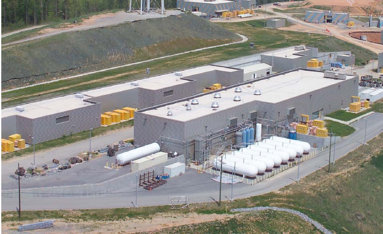
Fig. 5.5-7. Aerial view of the CHL and RF facilities.
