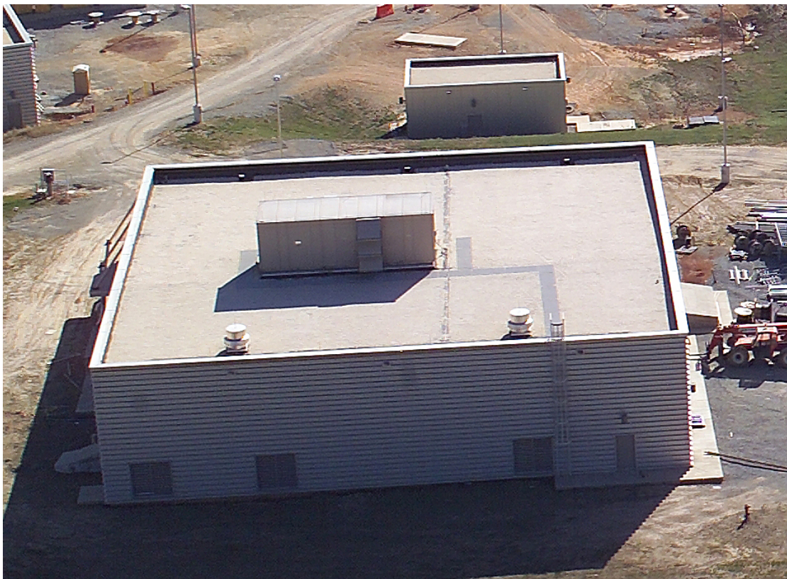
Fig. 5.5-11. Aerial view of the Ring Service Building.
