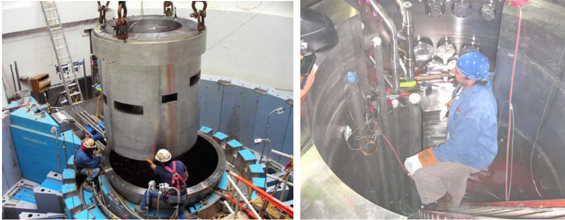
Fig. 5.2-30. Installation of lower outer reflector plug completed April 2005.
