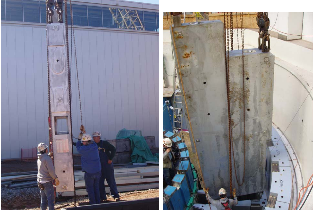
Fig. 5.2-48 Installation of a typical shutter.
