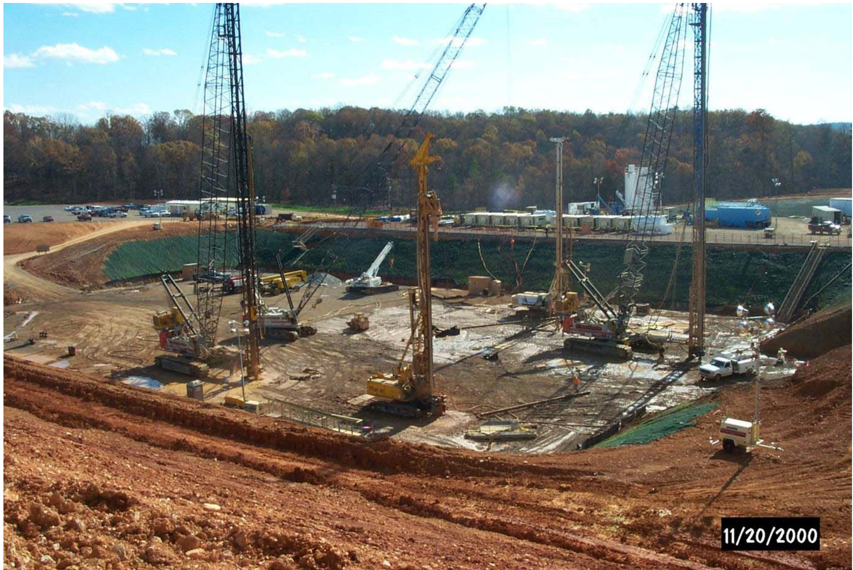
Fig. 5.5-13 Target Building construction--getting ready for concrete pilings.
