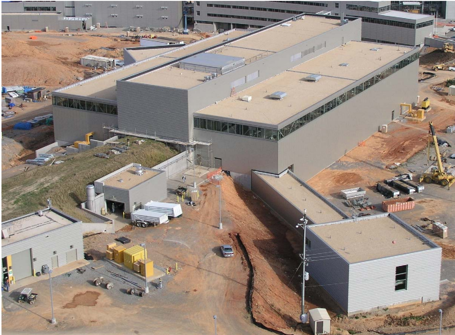
Fig. 5.5-17. Completed Target Building
