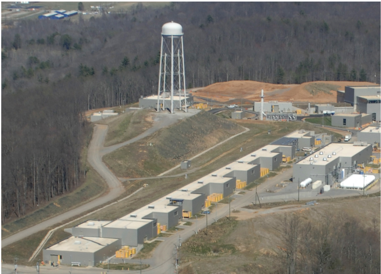
Fig. 5.5-3. Aerial view of the accelerator facilities.
