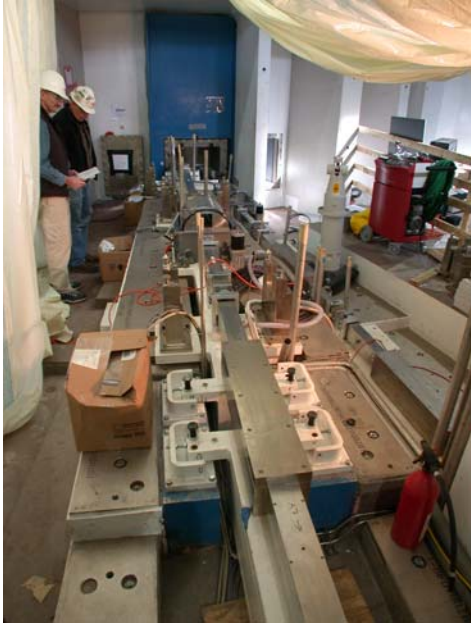
Fig. 5.3-14. Guide system and choppers: (a) guide system and secondary shutter installed, (b) choppers installed in guide openings and first shielding pieces in place.
