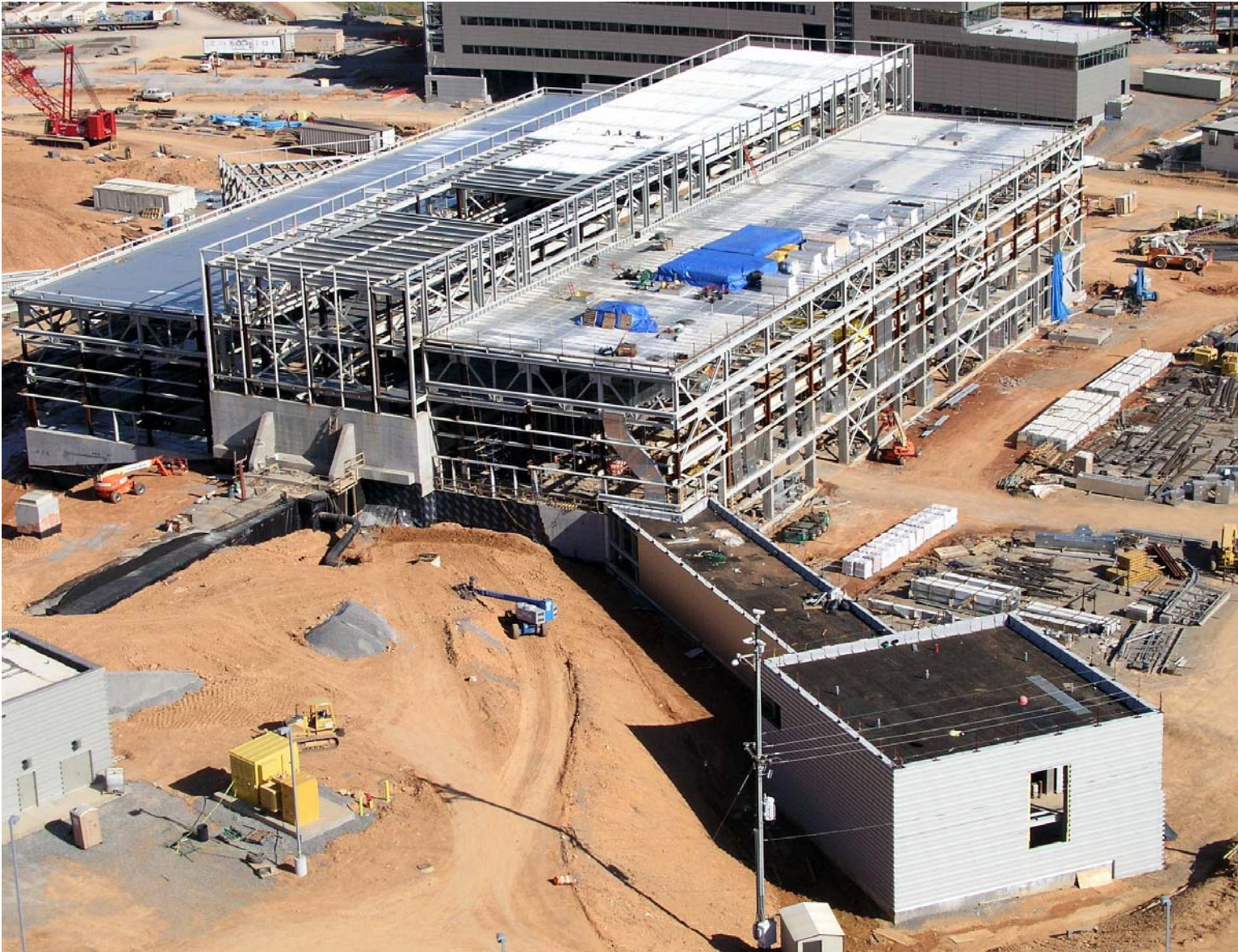
Fig. 5.5-16. Target Building and Backscattering Spectrometer Building construction.
