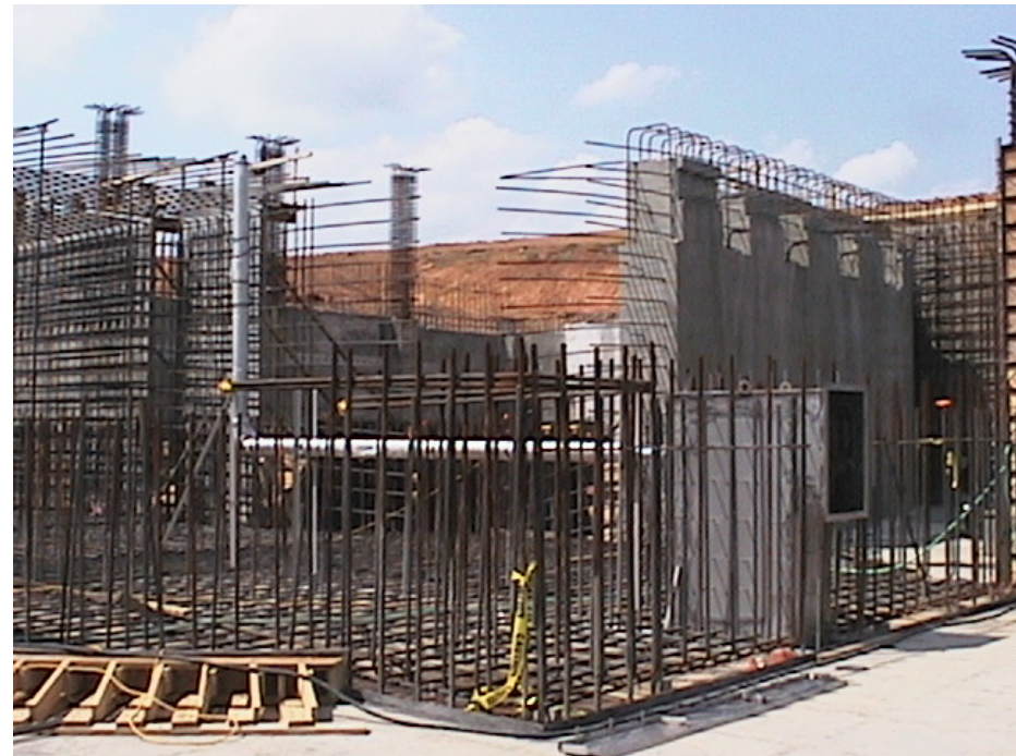
Fig. 5.2-45. Schematic diagram of bulk shielding liner spill drainage provision and initial installation.
