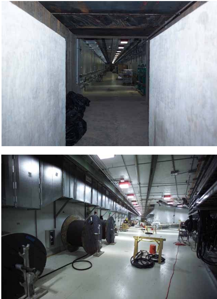
Fig. 5.5-10. HEFT, Ring, and RTBT tunnels.
