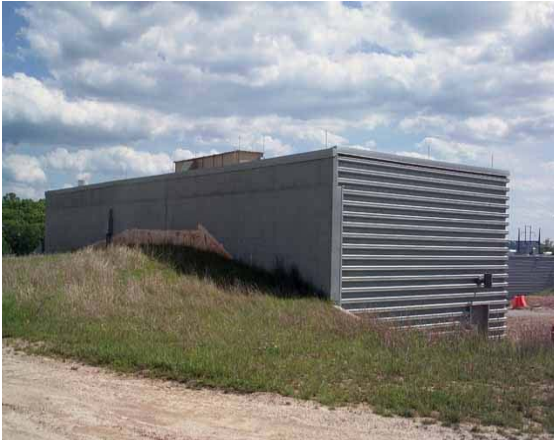
Fig. 5.5-9. Westward view of the RTBT Service Building.
