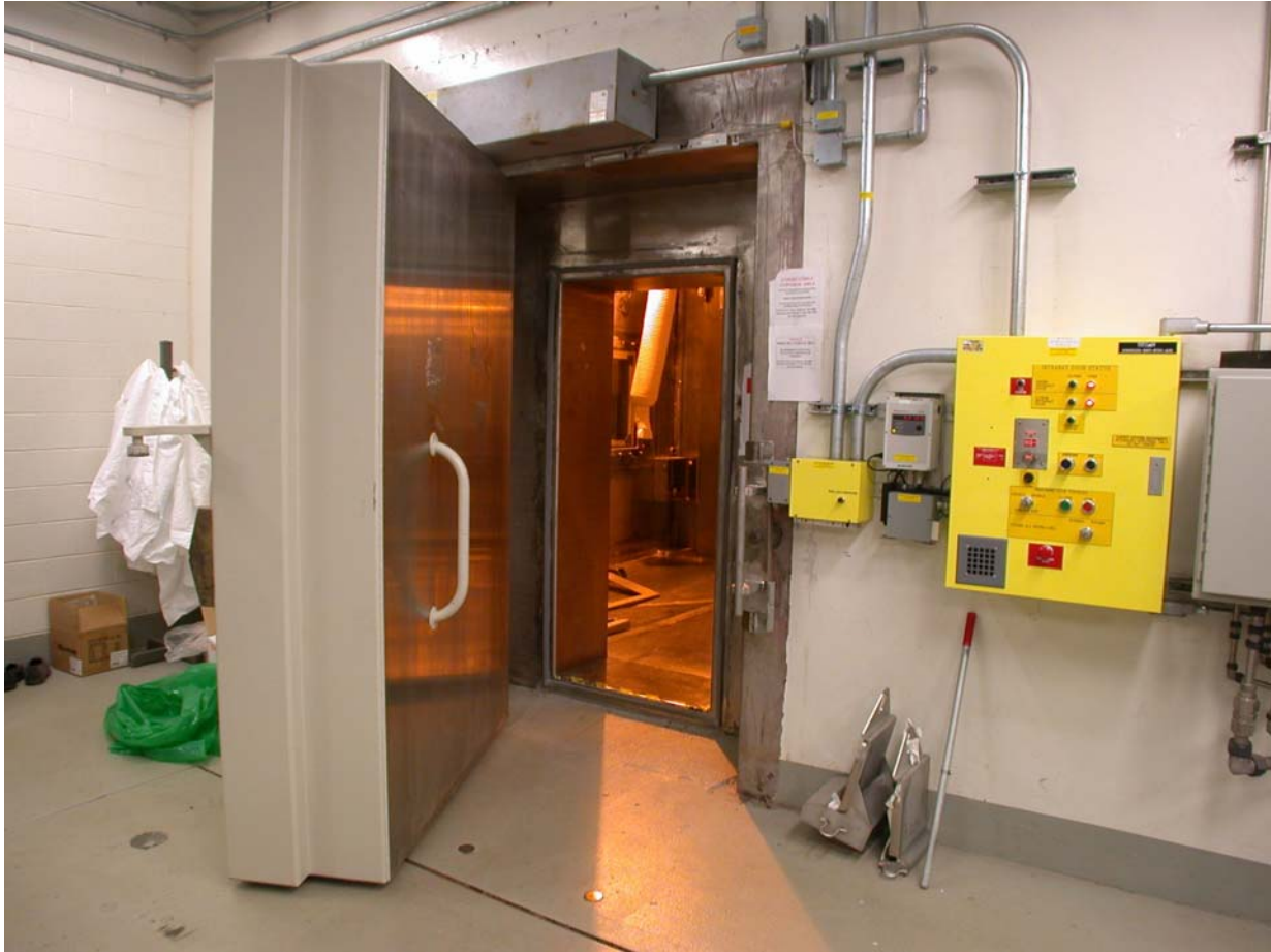
Fig. 5.2-67. Personnel door leading to transfer bay.
