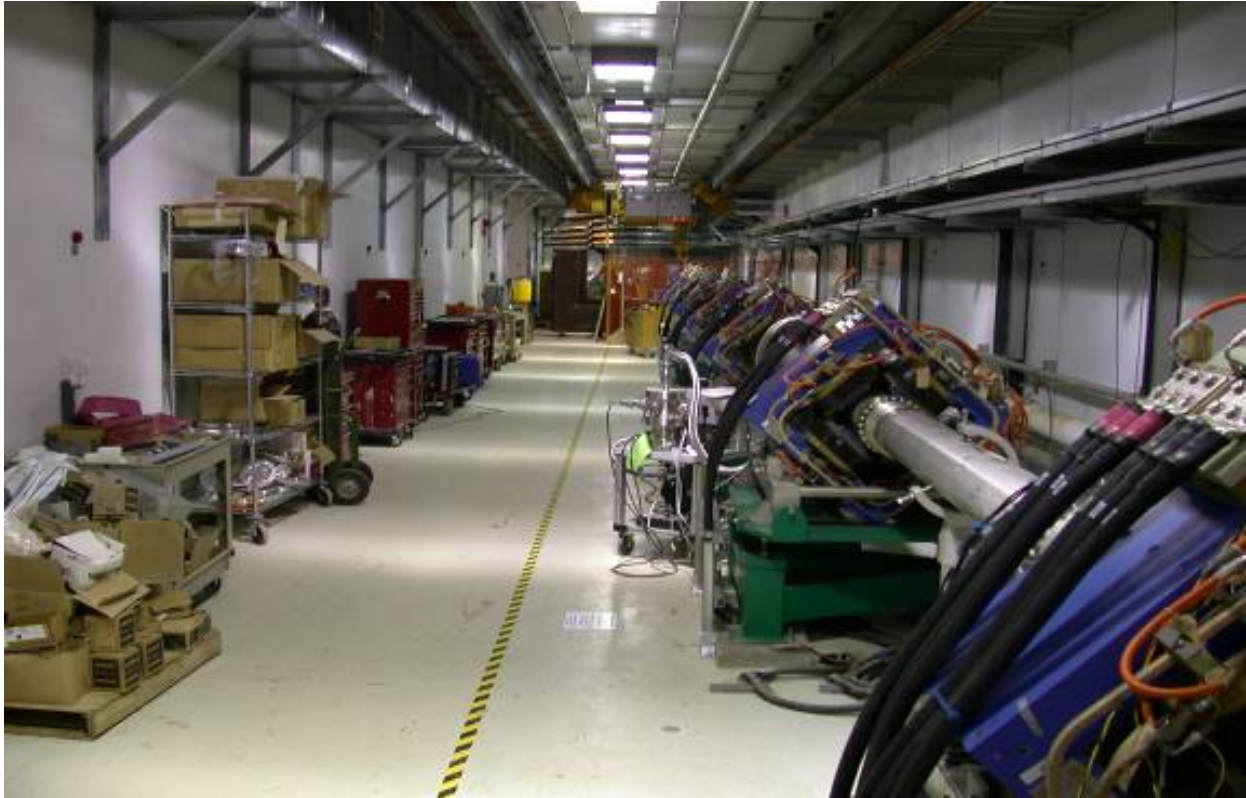
Fig. 5.1-27. Straight view into the RTBT tunnel toward the Target Building.
