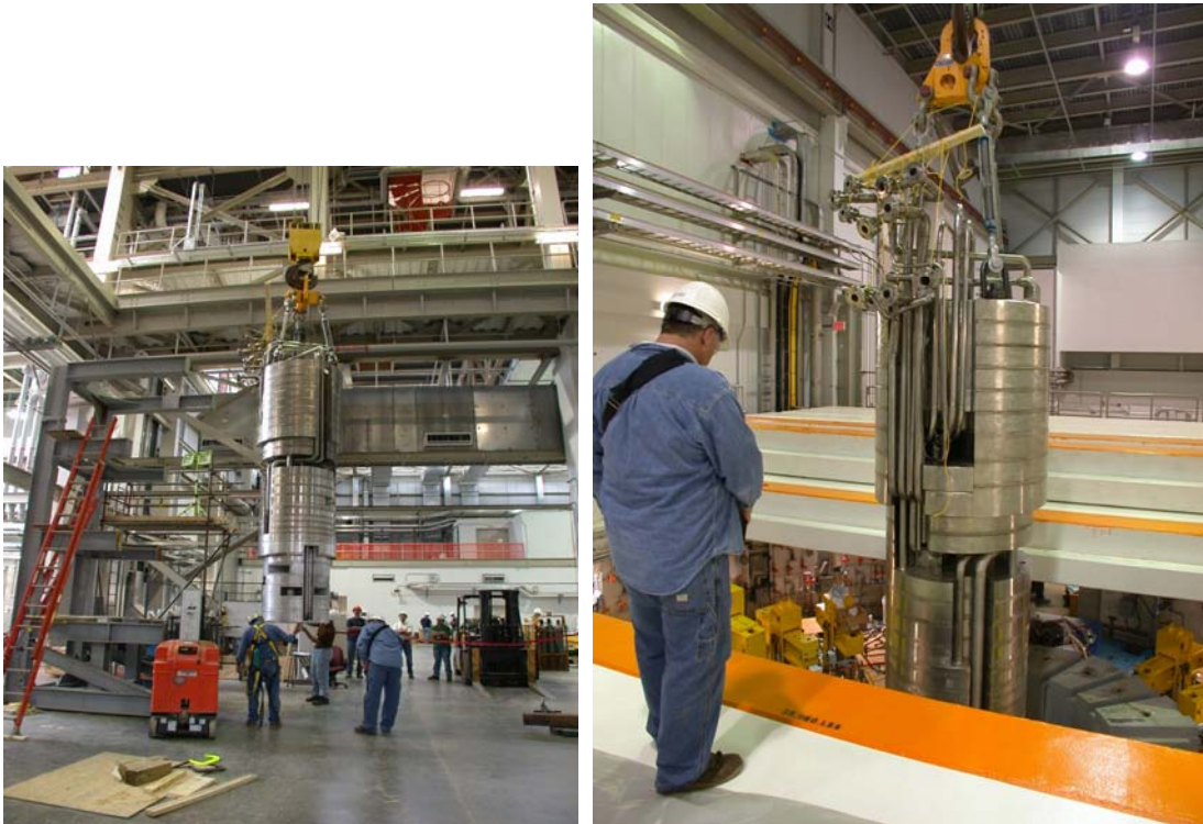
Fig. 5.2-31. Inner reflector plug just before installation.
