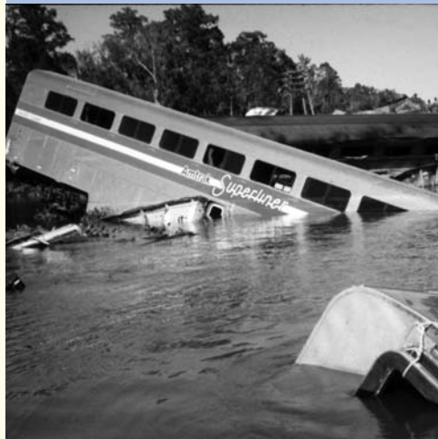
Forty-seven lives were lost when an passenger train derailed on a bridge and plunged into a bayou in 1993. Barges had previously hit the railroad bridge displacing the track.
