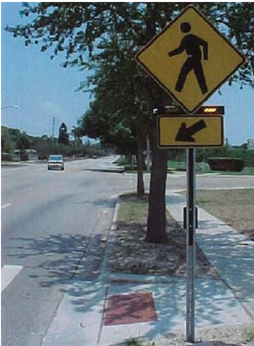
Example of RRFB with W1-2 sign and W16-7p plaque at crosswalk across uncontrolled approach. [Photo courtesy of City of St. Petersburg, Florida]
