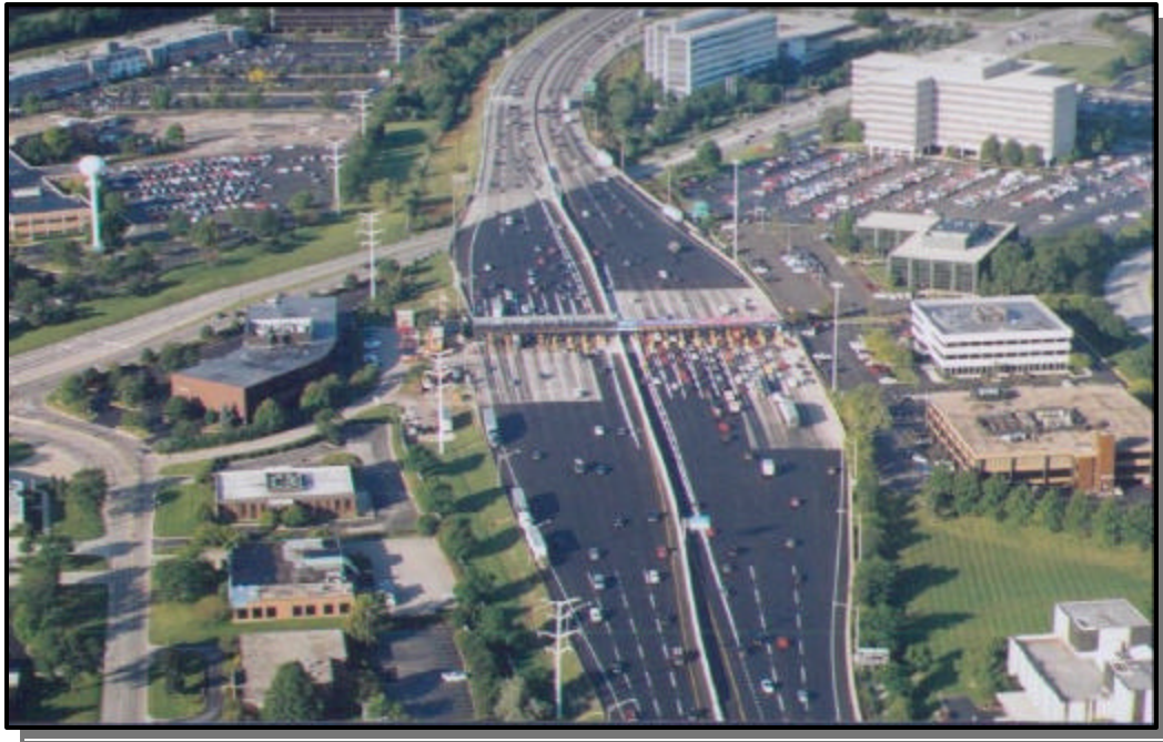
Exhibit 2-3 Mainline Barrier Plaza on the Illinois Tollway, I-88 York Road Plaza (1998)
