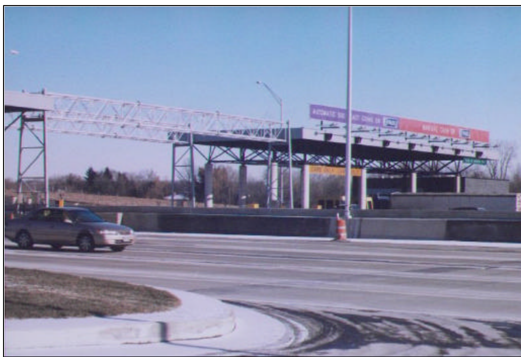
Exhibit 2-17 Illinois State Toll Highway Authority Access Way to Plaza Administration Building
