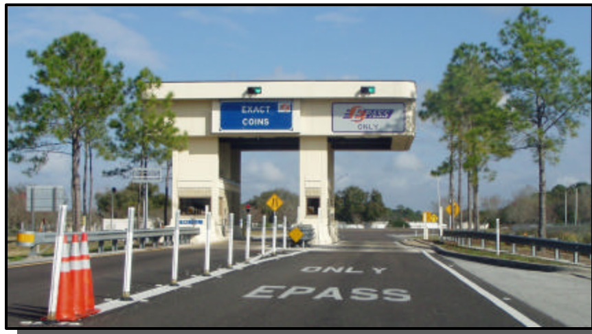
Exhibit 2-8 – Orlando Orange County Expressway Authority Ramp Toll Plaza with ETC Dedicated Lane Located to the Right (2004)
