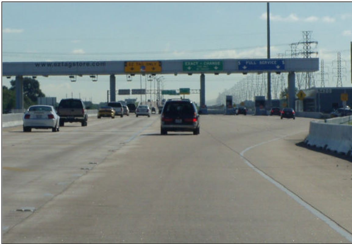
Exhibit 3-5 – Harris County Expressway Express Lanes and Conventional Plaza Lanes
