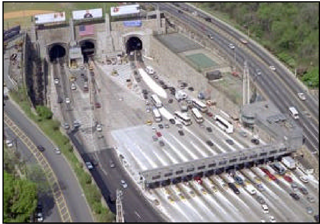
Exhibit 2-4 Tunnel Barrier Plaza on the New Jersey Side of the Lincoln Tunnel
