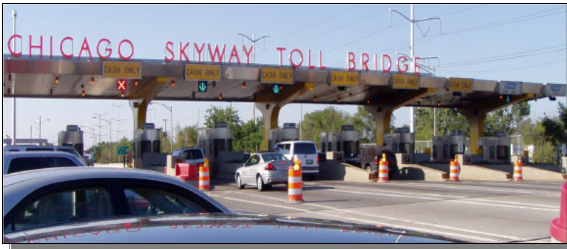
Exhibit 3-6 Chicago Skyway Bridge Canopy Signing
