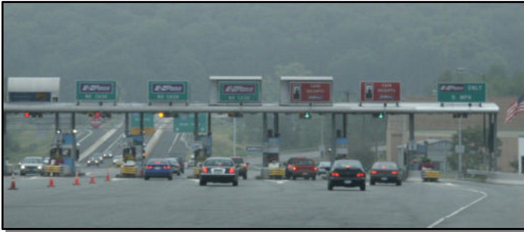
Exhibit 2-6 – New York State Thruway Plaza with Multiple ETC Dedicated Lanes Located to Left (ca. 2002)
