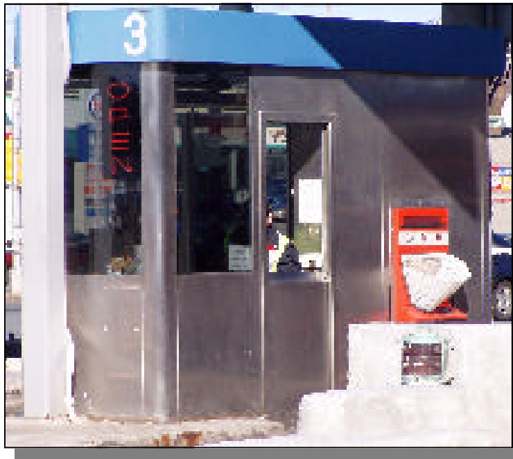
Exhibit 5-9 Halifax Dartmouth Bridge Commission Tollbooth/ ACM Combination
