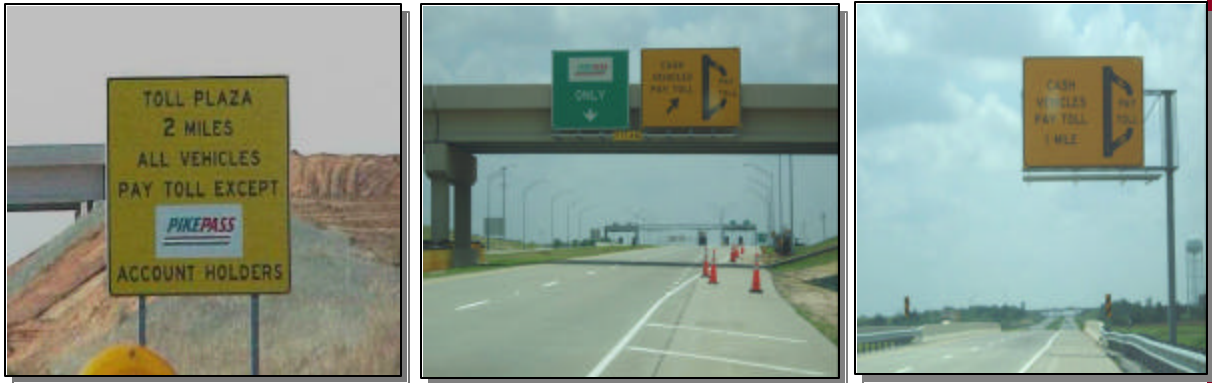
Oklahoma Turnpike Advance Toll Plaza Signing
