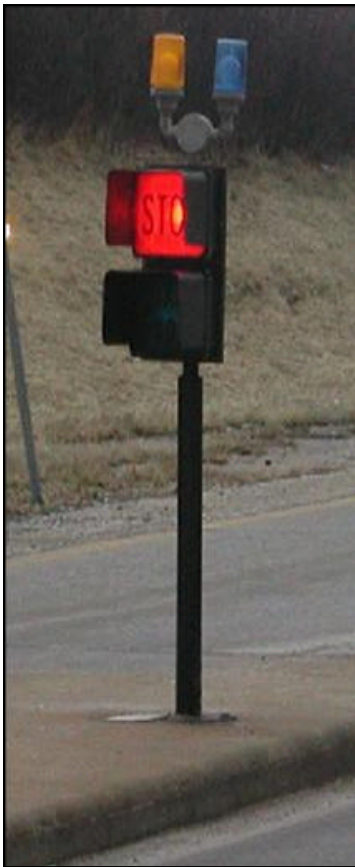
Exhibit 5-3 Illinois Tollway ITS w/I-PASS Acct. Status Lights and E-470 ITS w/Violation Alarm & Light (right)
