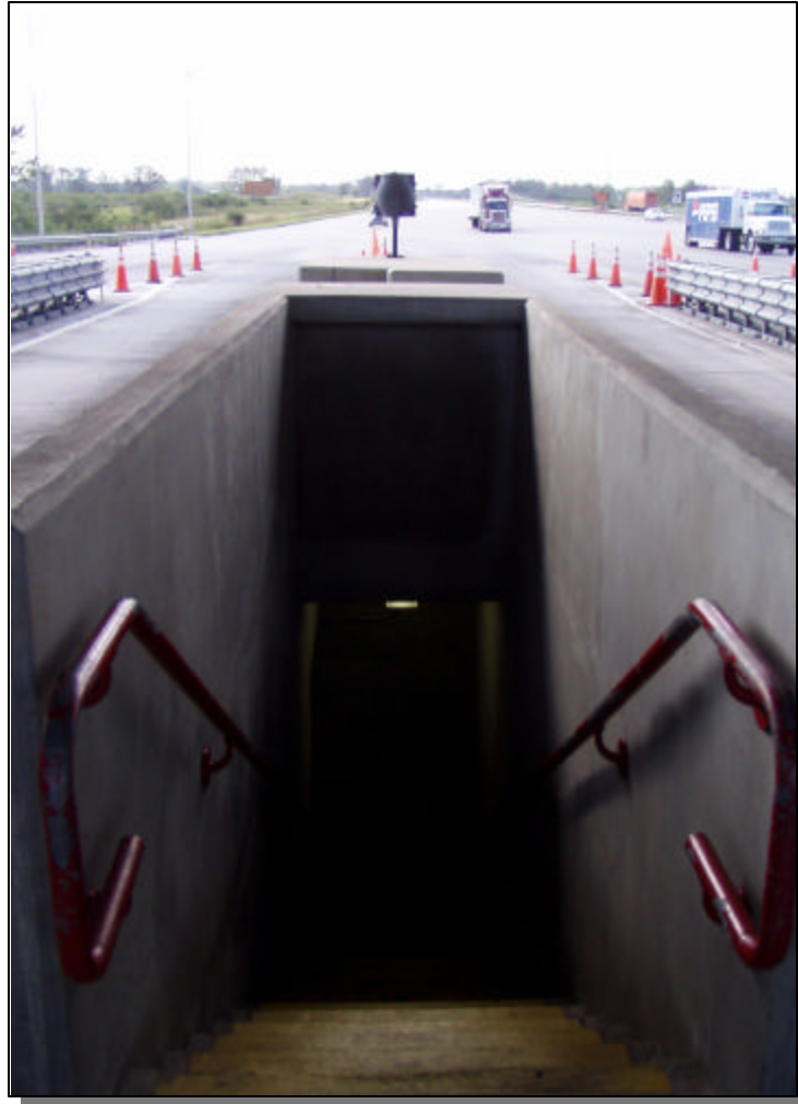
Exhibit 2-18 – Florida Turnpike Enterprise Stairwell to Tunnel for Toll Collection.
