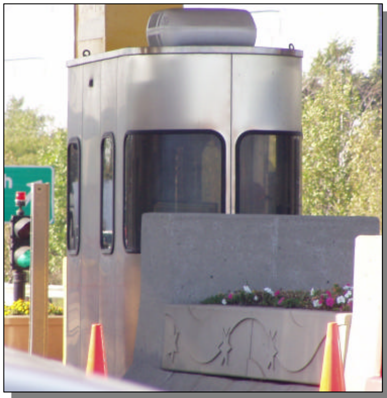
Exhibit 5-8 Chicago Skyway Bridge Tollbooth and Planter
