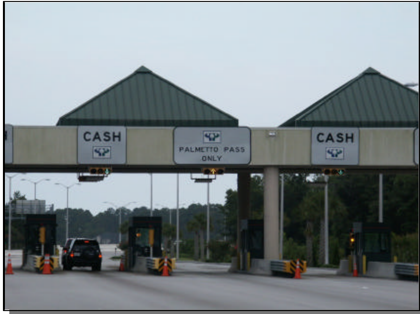
Exhibit 2-7 – Hilton Head Island Toll Plaza with a Dedicated Lane Located in the Middle (ca. 2002)
