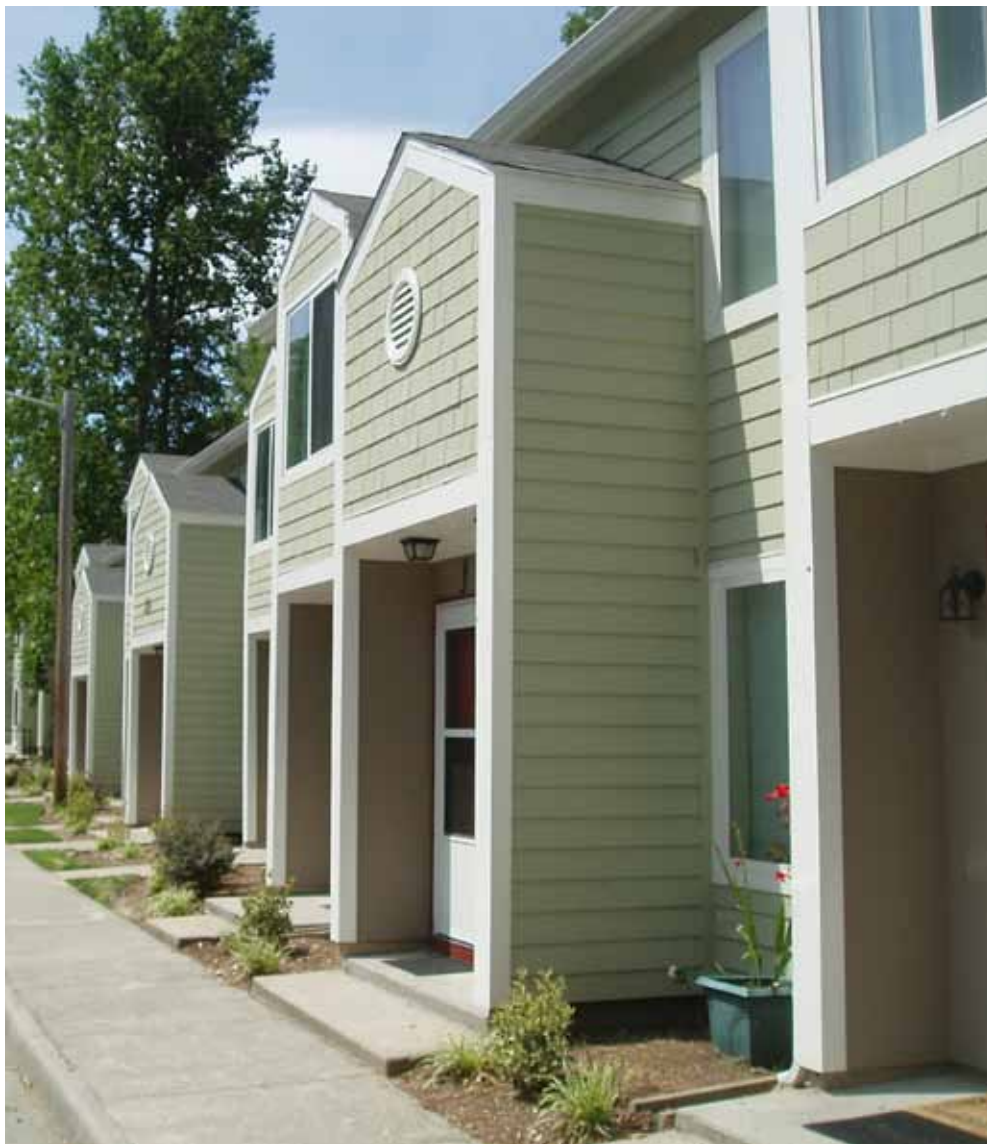
Community Housing Partners recently completed a “green” renovation of Yorktown Square II, which provides housing to low-income residents of Yorktown, Virginia.
