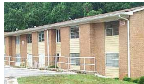
Before: Flat Shoals apartments, in Atlanta, Georgia, before renovations began.
