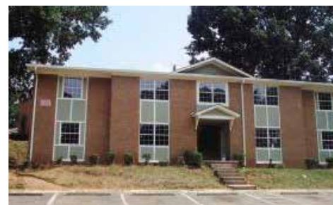
After: The rehabilitated apartments of Flat Shoals.
