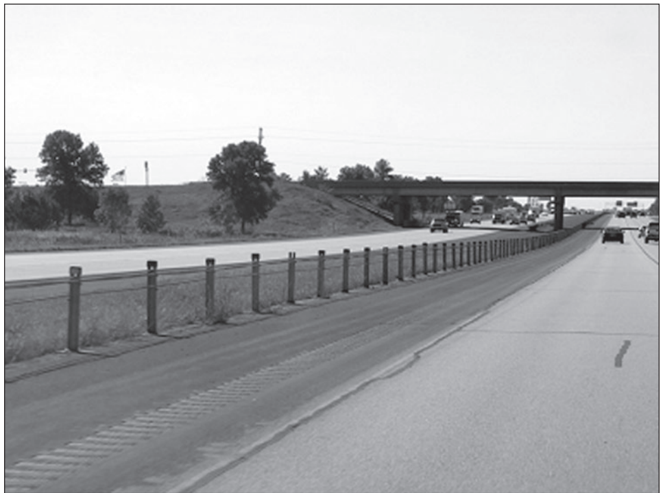
Figure 4: Rumble Strips and Cable Median Barriers in Iowa Designed to Keep Drivers on the Road and Reduce Head-on Collisions
