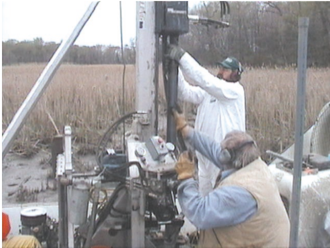
(A) Coring with the hoverprobe
