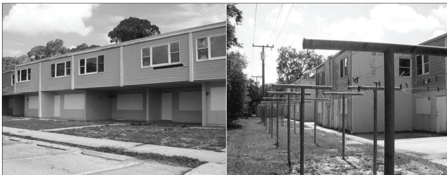
Figure 6: Front and Back View of Vacant Rental Units Scheduled for Demolition by Venice Housing Authority
