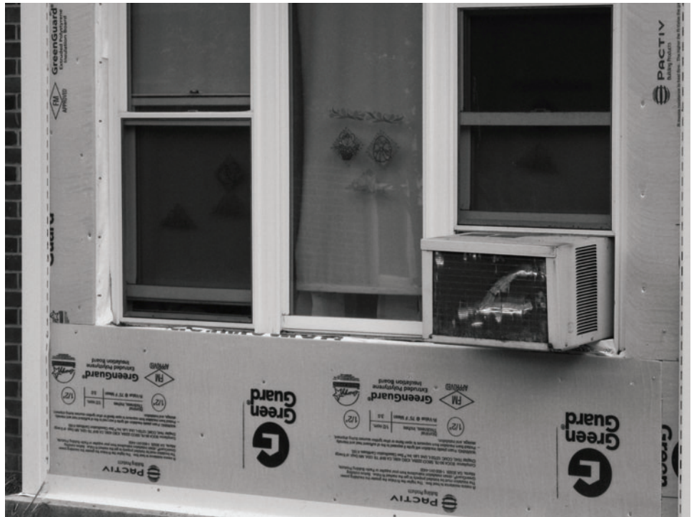
Figure 6: In-Progress Siding Installation Using Recovery Act Funds, Rahway, New Jersey
