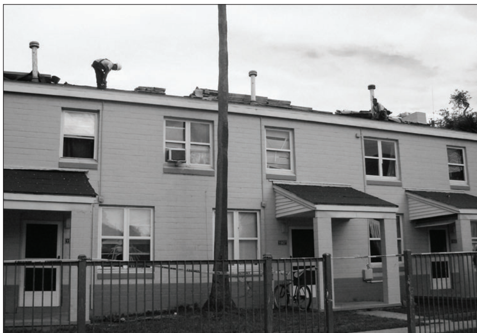
Figure 7: Workers Repairing Roof at Public Housing Development for Tampa Housing Authority
