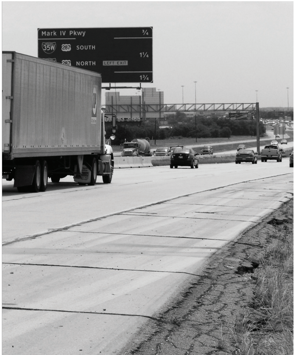
Figure 3: Fort Worth District Roadway Resurfacing
