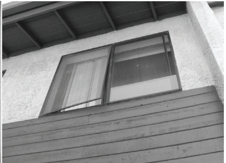
Window soon to be replaced with energy-efficient, double-pane windows in Ventura.
