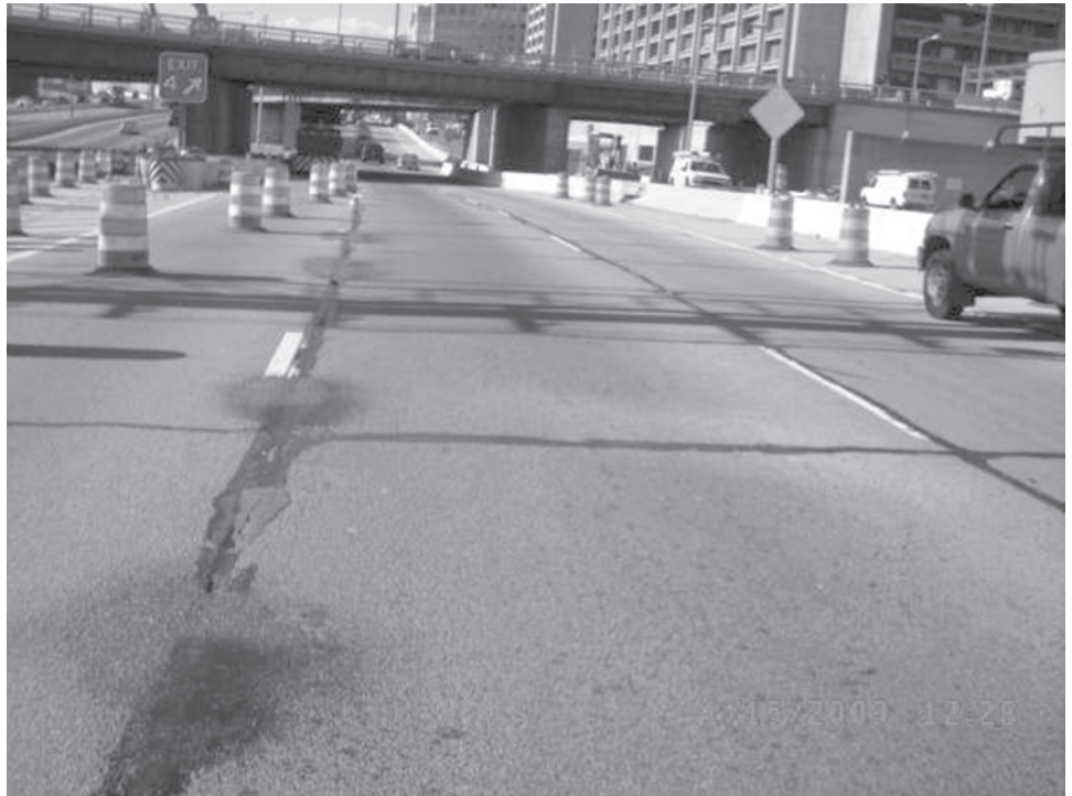
Figure 2: Portion of Interstate 395 in Southwest Washington before Repaving, January 15, 2009
