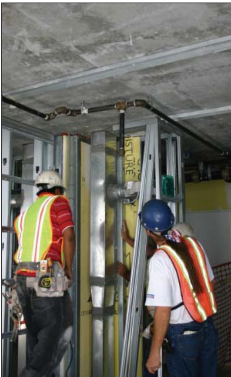
Inside a room on the 3rd floor of Pavilion A.
