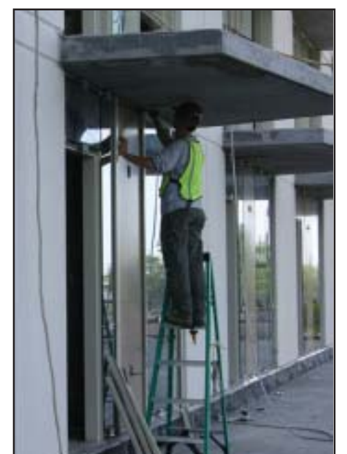
Pavilion A, 2nd Level, west side.
