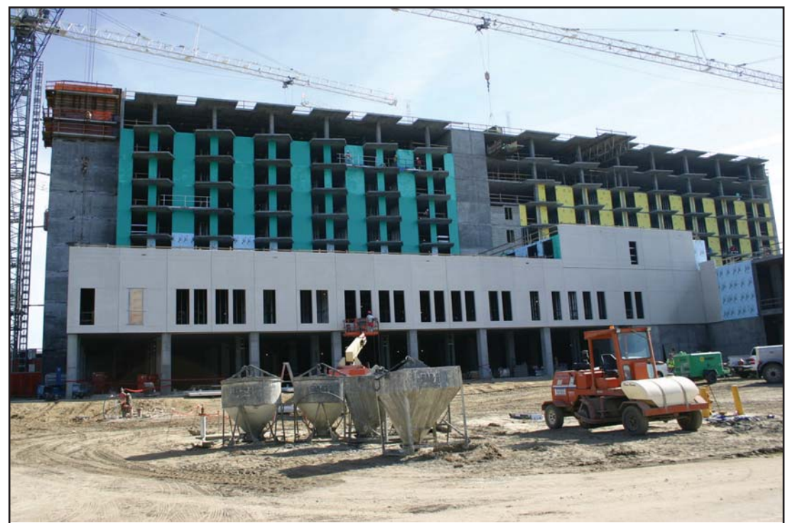
The north west side of Pavilion A.
