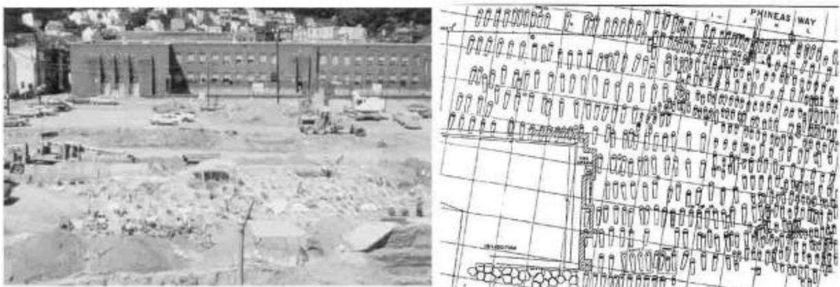
Excavation Site and Layout of Graves
