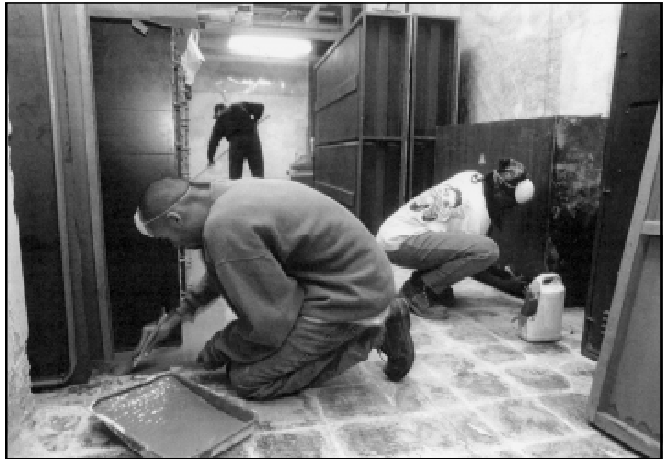
Work crew members paint a corridor at a local university.
