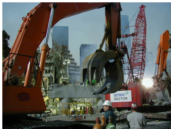
Heavy equipment in use at Ground Zero
