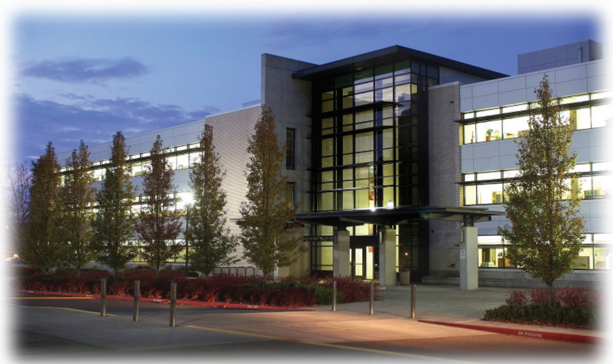
OHCS Headquarters, the North Mall Office Building, Salem
