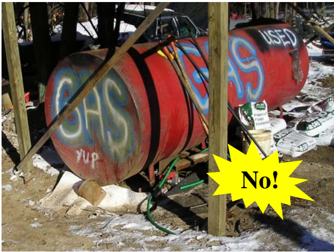
Even though this tank is labeled clearly and sheltered by a roof as required, it is not correctly installed. It must also be placed inside a secondary containment device and be surrounded by a concrete refueling pad.
