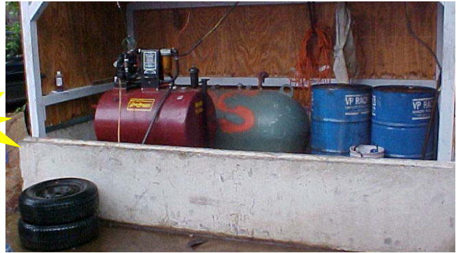
Put the containers inside a secondary containment device, such as half a concrete septic tank or a steel box. Shelter the entire structure from precipitation.
