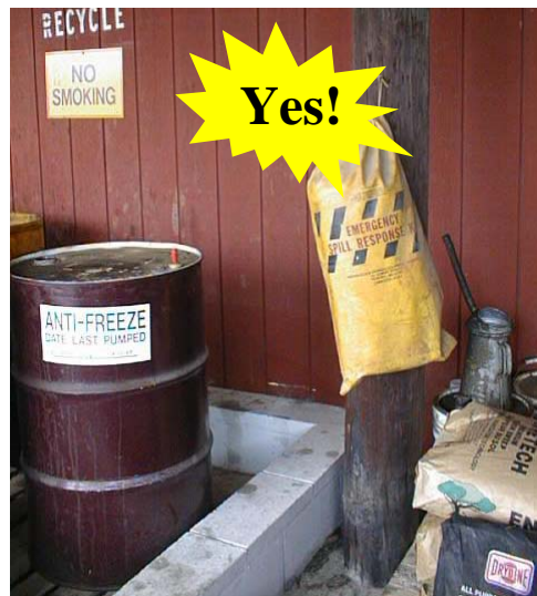
Keep a spill kit near all area where fluids are handled or stored.
