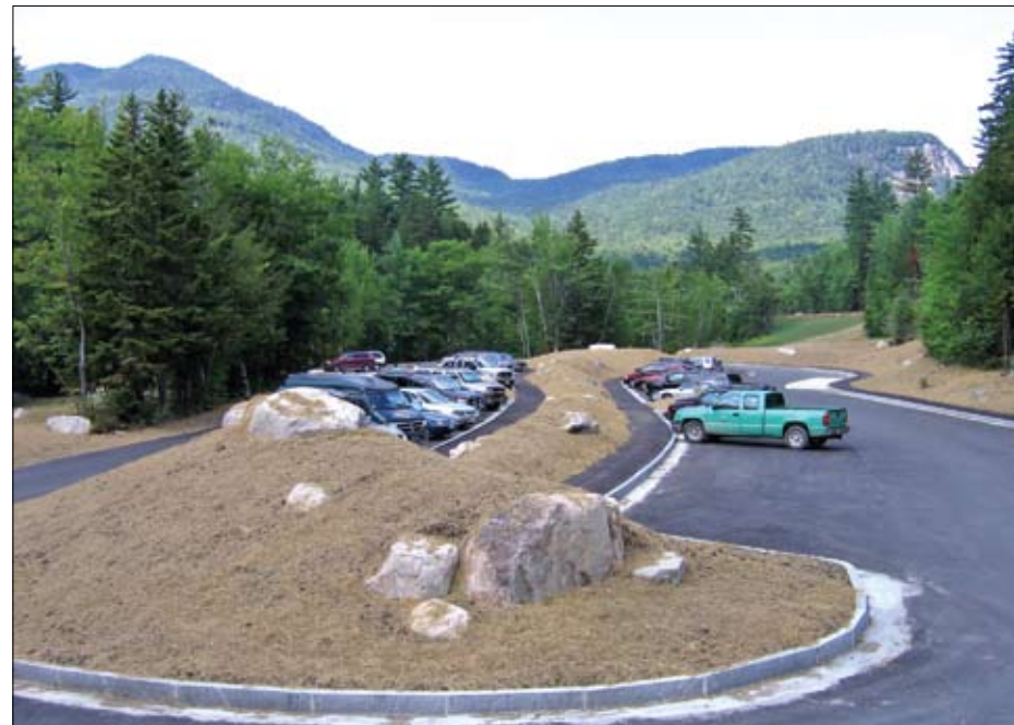
Rocky Gorge Recreation and Scenic Area Renovation (Ken Allen)
