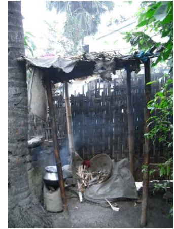
An outdoor kitchen Photo credit: Winrock
