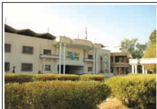
The Kirkuk Government Building, in downtown Kirkuk, is the center of political activity and governance supported by the 116 BCT, in north central Iraq.
