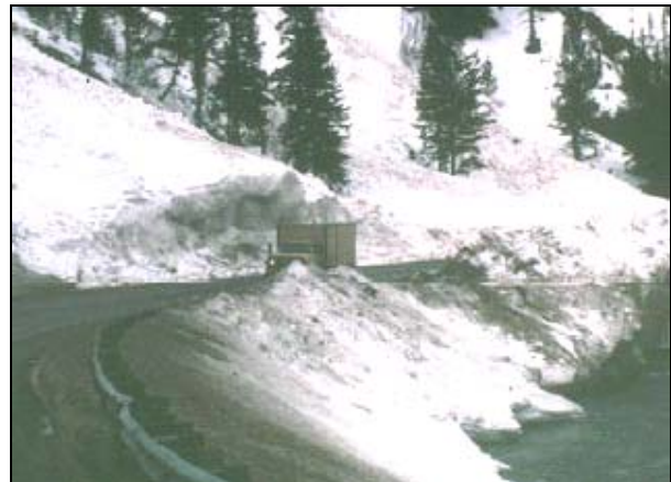
Wyoming DOT Avalanche Warning System Location
