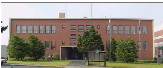
Lincoln County Courthouse, Newport
