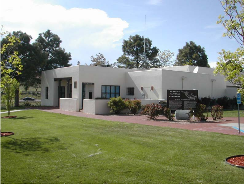
Photo 1: Looking at the Santa Fe National Cemetery administration/visitors center building.
