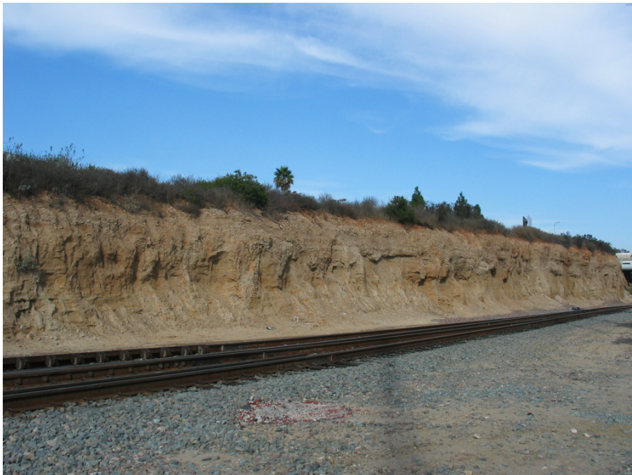
b. View from railroad tracks at the northeastern edge of the site looking northeast.
