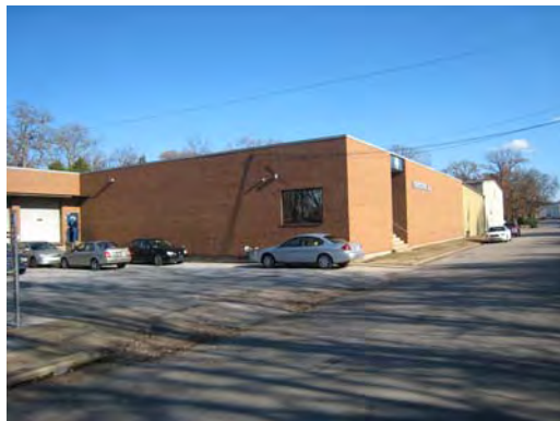
PHOTO 11. Fabricators Inc. (Parcel ID – 146P C 014)
