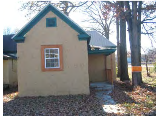
PHOTO 4. Typical residential lot within area of investigation (Parcel ID – 146P B 002)
