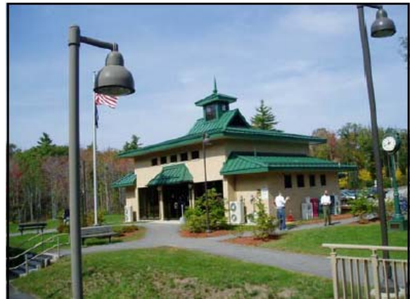
Wells Transportation Center
