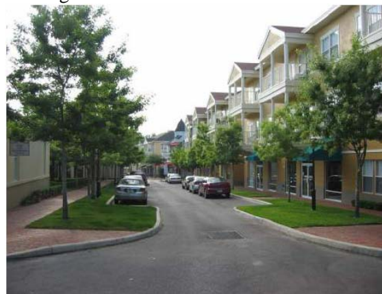
Exhibit 24: Narrow travel lanes and on-street parking help reduce runoff.
