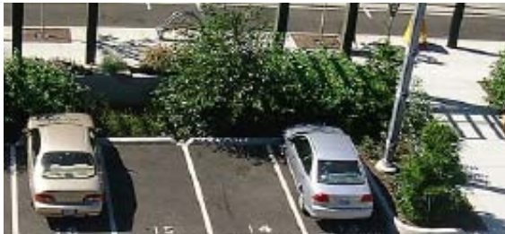
Exhibit 26: This parking lot retrofit (above) and parking lot basin (right), demonstrate how adding infiltration basins requires little space and adds more greenery to the streetscape.
