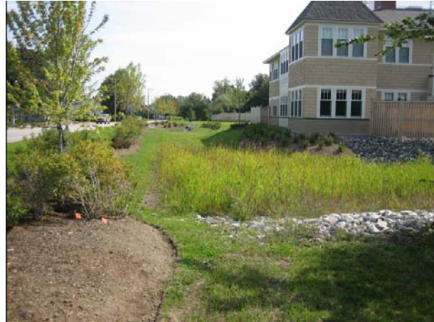
The town of Wells has experience with infiltration approaches. The new medical center on Rt. 109 has a good example of a swale that manages stormwater on-site.
