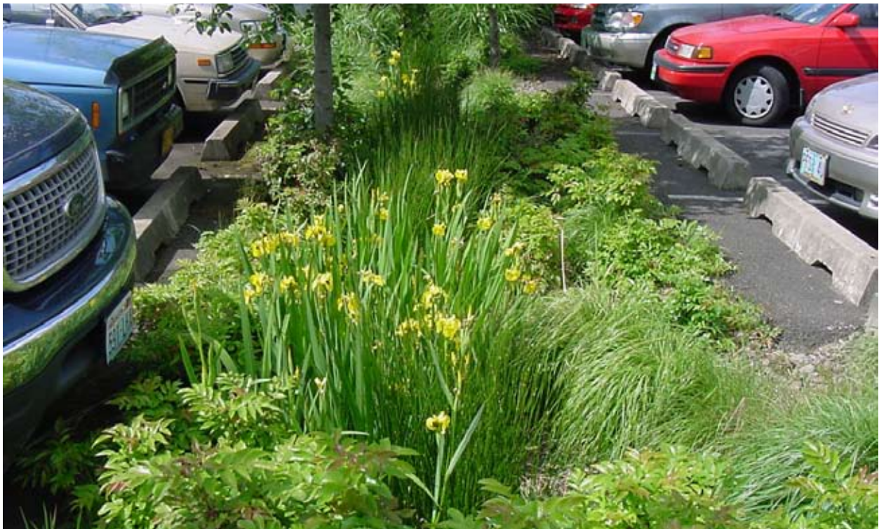
Figure 5-69: This parking lot in Portland, Oregon was built with a center median stormwater swale.
