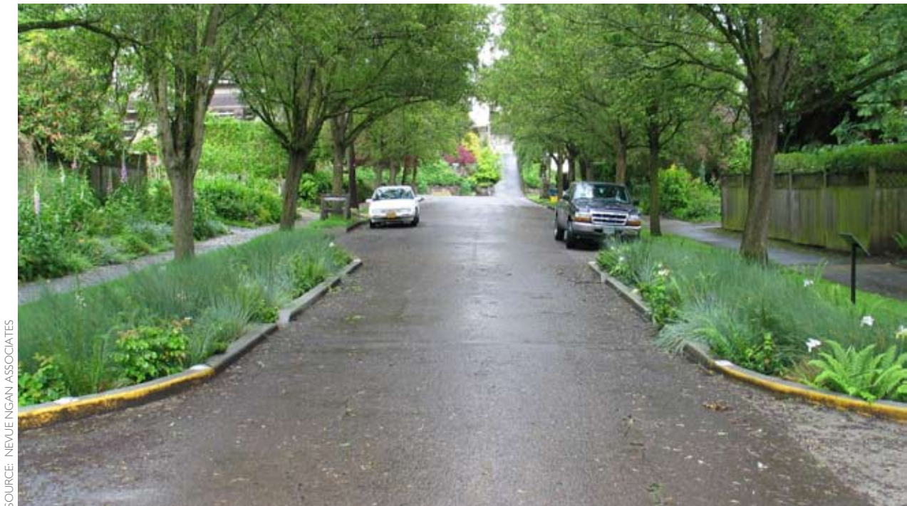
Figure 5-9: A pair of stormwater curb extensions used in a residential street's parking zone in Portland, Oregon.
