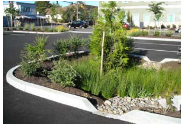
Figure 5-72: This parking lot manages a portion of its stormwater runoff with multiple stormwater planters.
