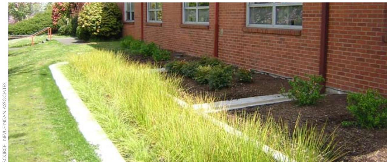
Figure 5-76: Disconnected downspouts at a school site in Portland, Oregon convey water into nearby infiltration planters.
