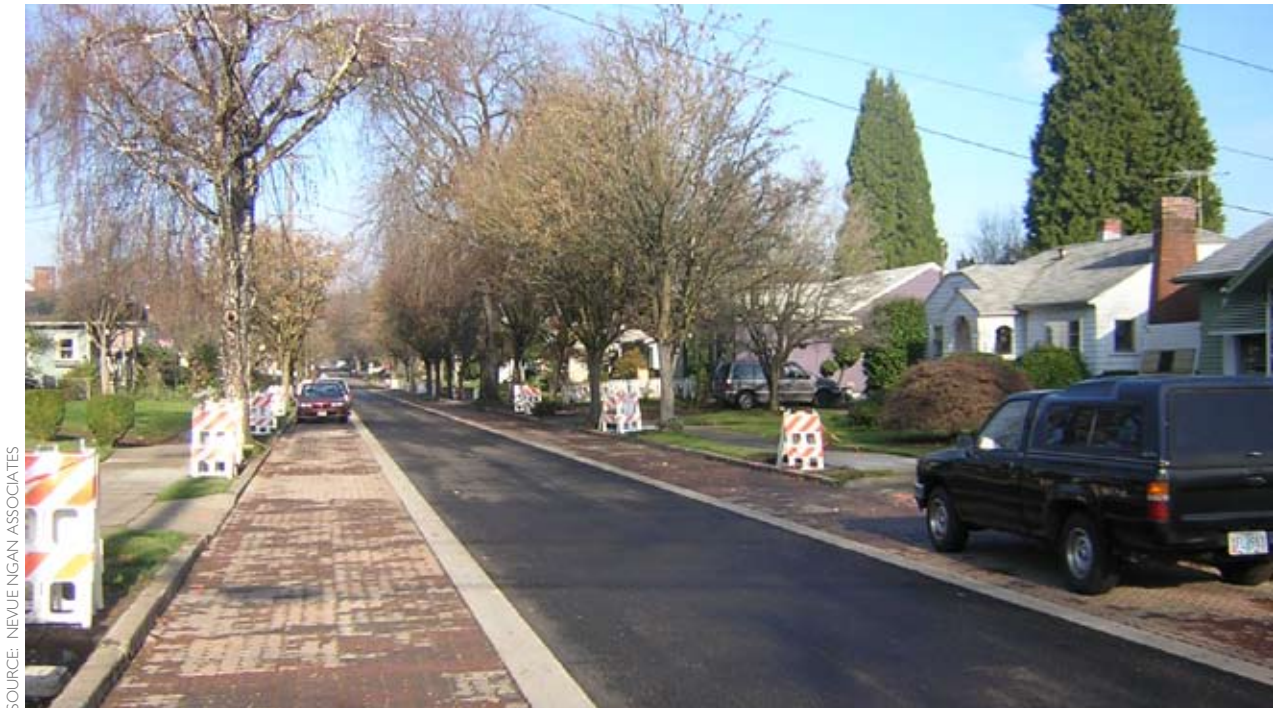
Figure 5-21: Pervious paving used in a residential street's parking zone. Notice the visual "narrowing" of the street.
