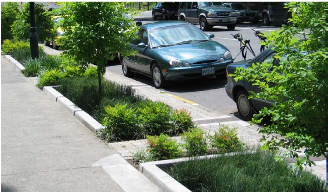
Figure 5-29: Stormwater planters used along a downtown street. Space should be allocated for people to get in and out of their vehicles and access the sidewalk.
