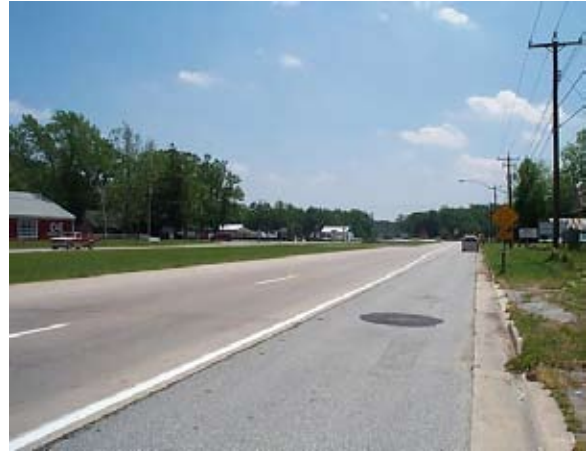
Figure 5-52: EXISTING: This arterial street in Lewes, Delaware has an extra wide shoulder that could be used more efficiently.
