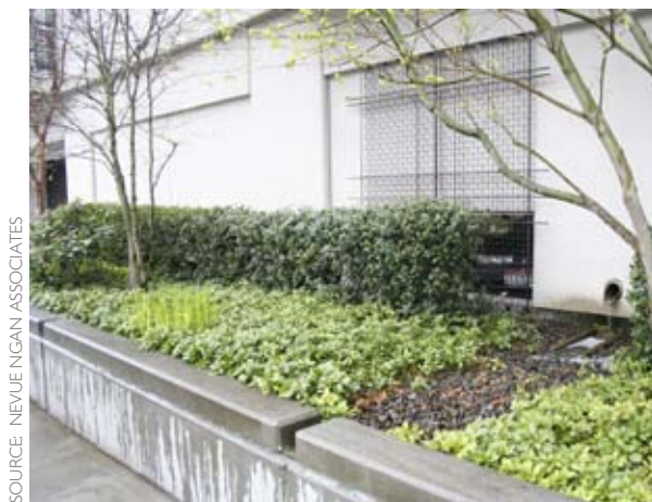
Figure 5-75: An infiltration planter along a building in Portland, Oregon manages stormwater runoff.
