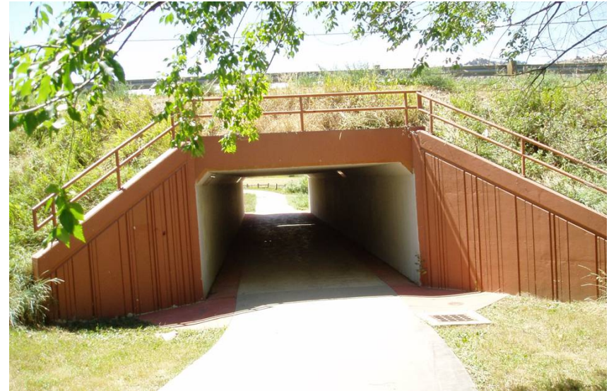
Figure 40: Grade separated crossing, Boulder
