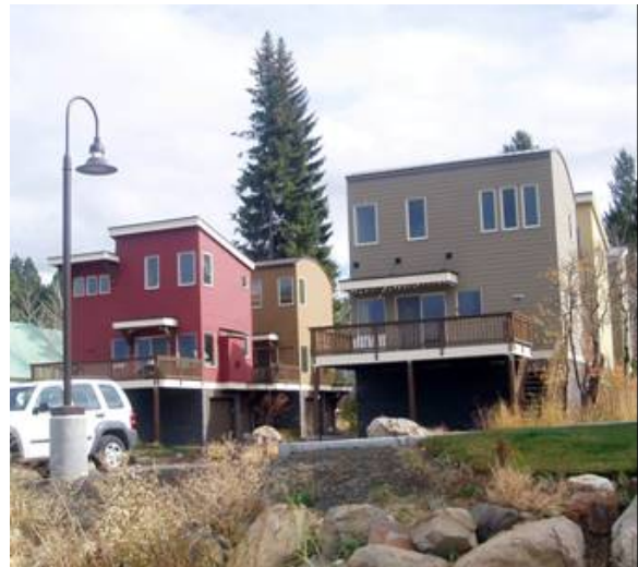
Figure 16: Local multi-story buildings illustrate possibilities for compact, appropriate design.
