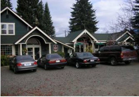
Figure 13: An example of ground-floor retail with a second floor that could be used for office or apartment. Buildings like this, located closer to the street, would provide a sense of place.
