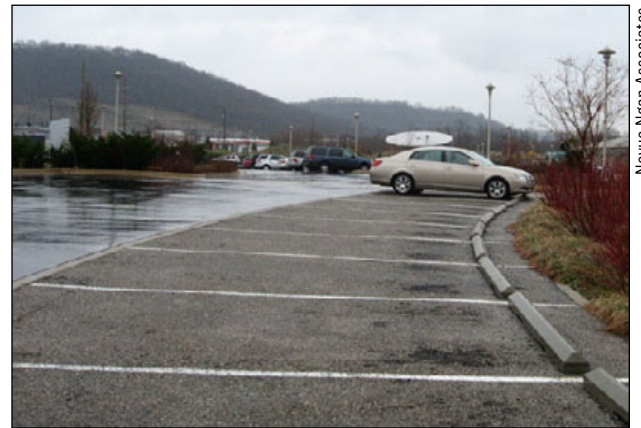
Figure 45. There is no wet sheen on the pervious asphalt in the parking stalls in this parking lot, compared to the conventional asphalt paving in the drive aisles.
