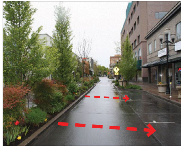
Figure C-22. An existing landscaped median on a crowned street can be a difficult retrofit project because water flow is directed away from the middle of the street.
