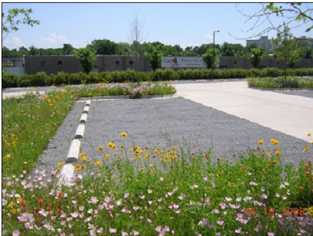
Figure 50. Reinforced gravel paving in parking stalls.
