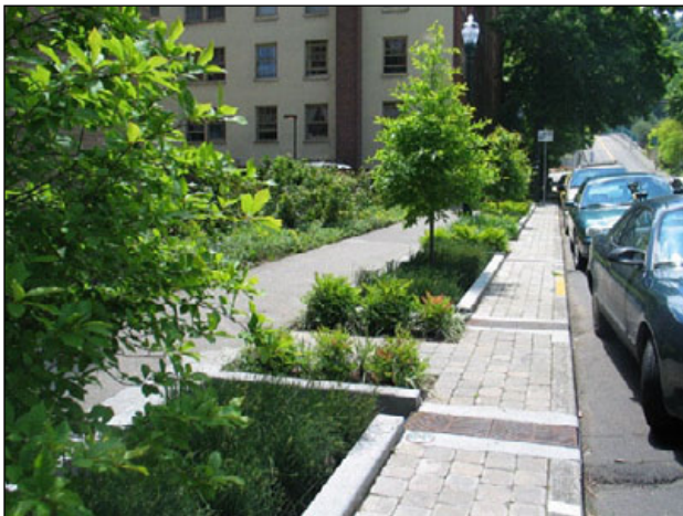
Figure 100. Stormwater planters along a downtown street allow on-street parking to be retained. A strip of pervious pavers allows access to parked cars.
