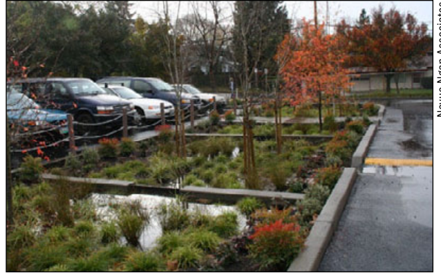
Figure 93. Parking lot swale with curb cuts and a speed bump used to direct stormwater flow.
