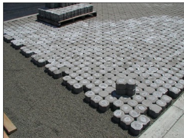
Figure 48. Interlocking concrete unit pavers create gaps between adjoining pavers, allowing water to soak into the ground.
