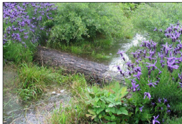
Figure C-29. Log check dam.
