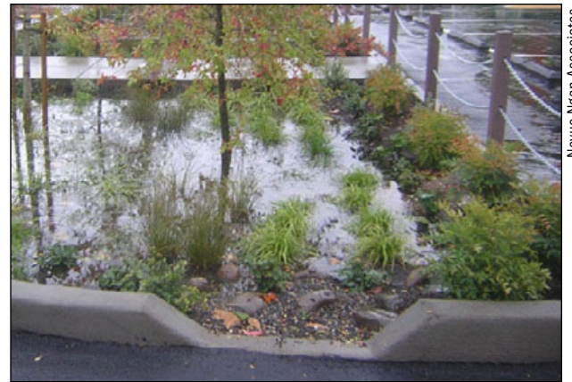
Figure C-32. A curb cut serves as the only overflow in this infiltration garden.
