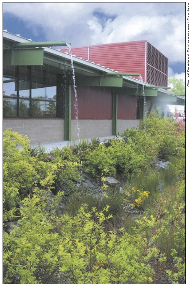
Figure 121. An infiltration garden treats roof runoff from a commercial building.
