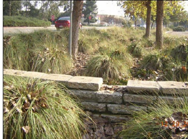
Figure C-27. Stacked concrete check dam.
