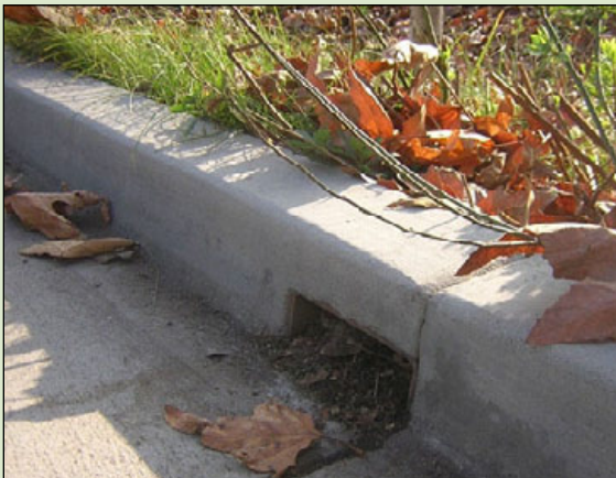
Figure C-14. Notched curb cut.
