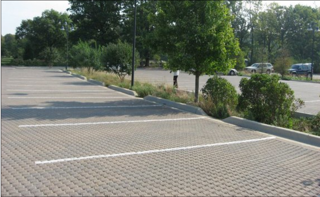
Figure 46. Pervious pavers in a parking lot application. Any overflow from the pervious pavers drains into a swale.
