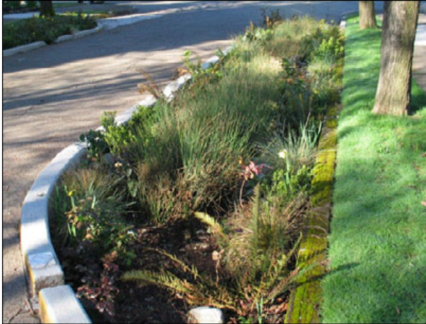
Figure C-23. Typical sediment forebay.
