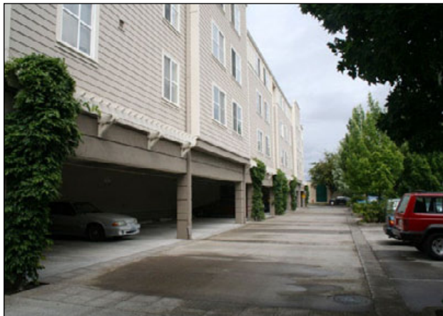
Figure 30. This apartment complex allows cars to park under the building's second floor, which uses the site more efficiently.
