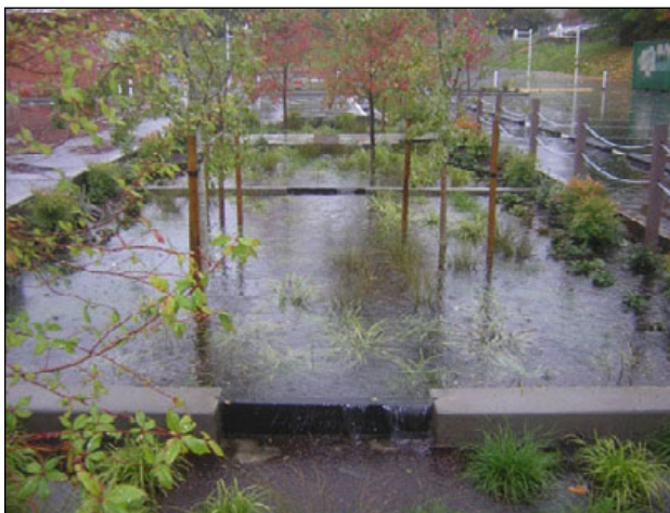
Figure C-26. Concrete check dam with an adjustable weir.
