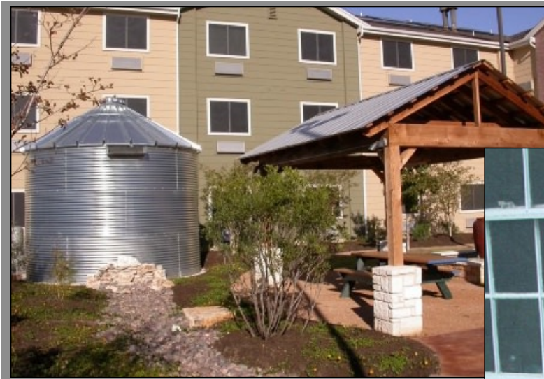
Figure 64. Large-scale commercial cisterns can hold large volumes of rainwater for reuse in toilets and irrigation systems.
