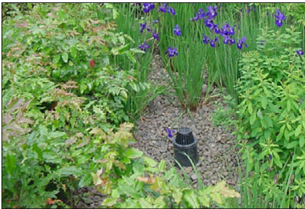
Figure C-31. A small-scale overflow stand pipe.
