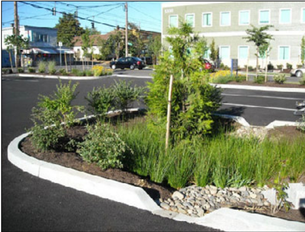
Figure 109. This parking lot manages a portion of its stormwater runoff in multiple landscape islands.
