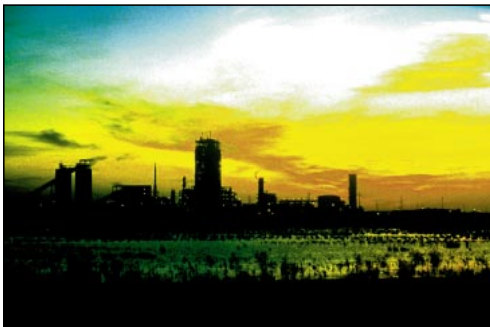
Dawn arrives over the reclaimed wetlands surrounding the Tampa Electric Integrated Gasification Combined-Cycle Project
