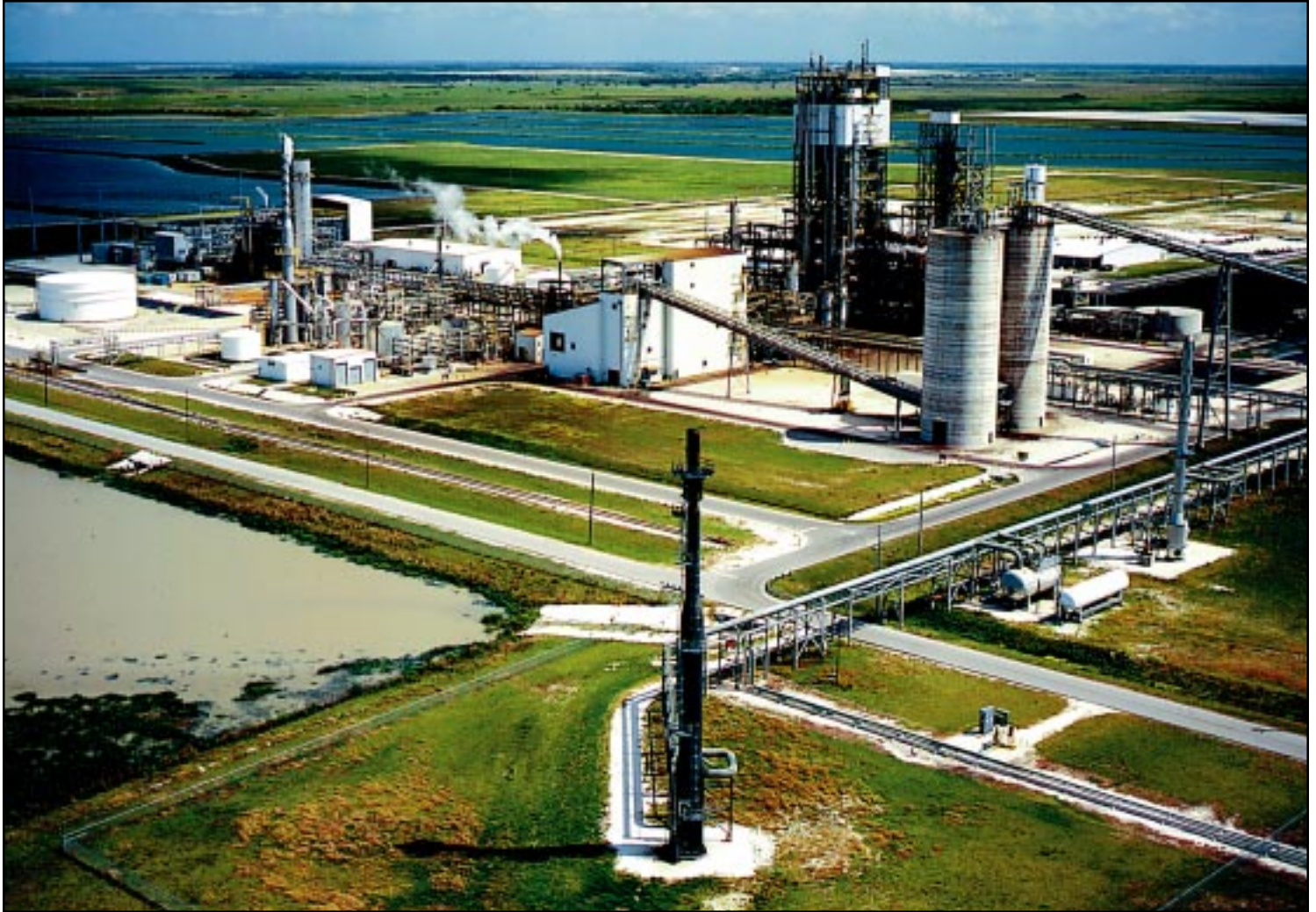
Aerial view of Polk Power Station
