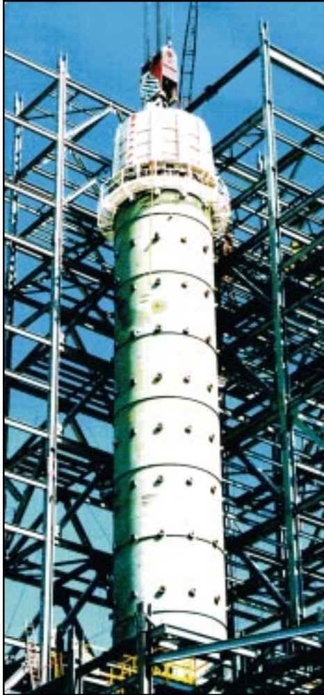
Installation of radiant syngas cooler
