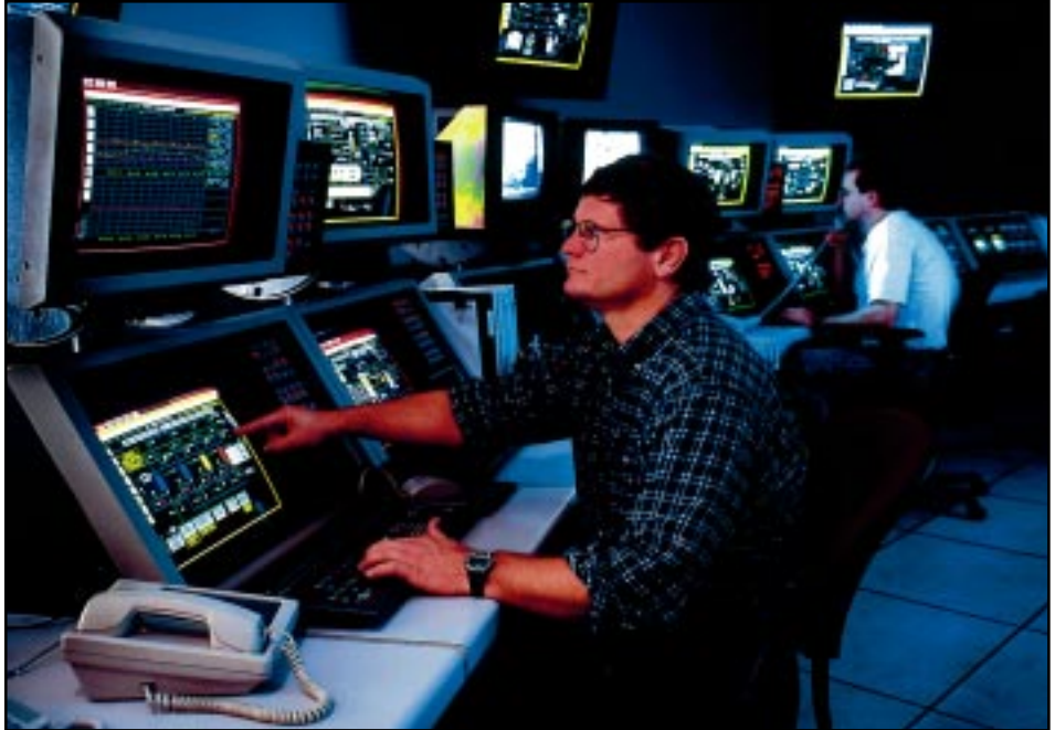
Polk Power Station control room
