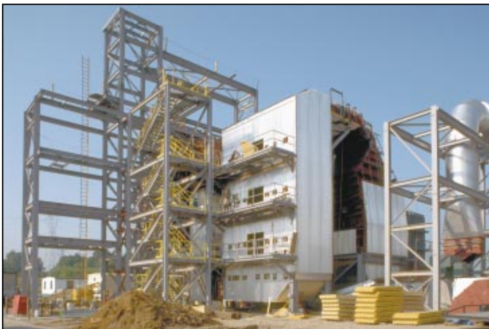
SNOX™ SCR reactor.
