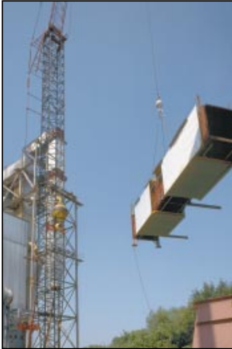
Duct section being hoisted into place during SNOX™ technology installation.
