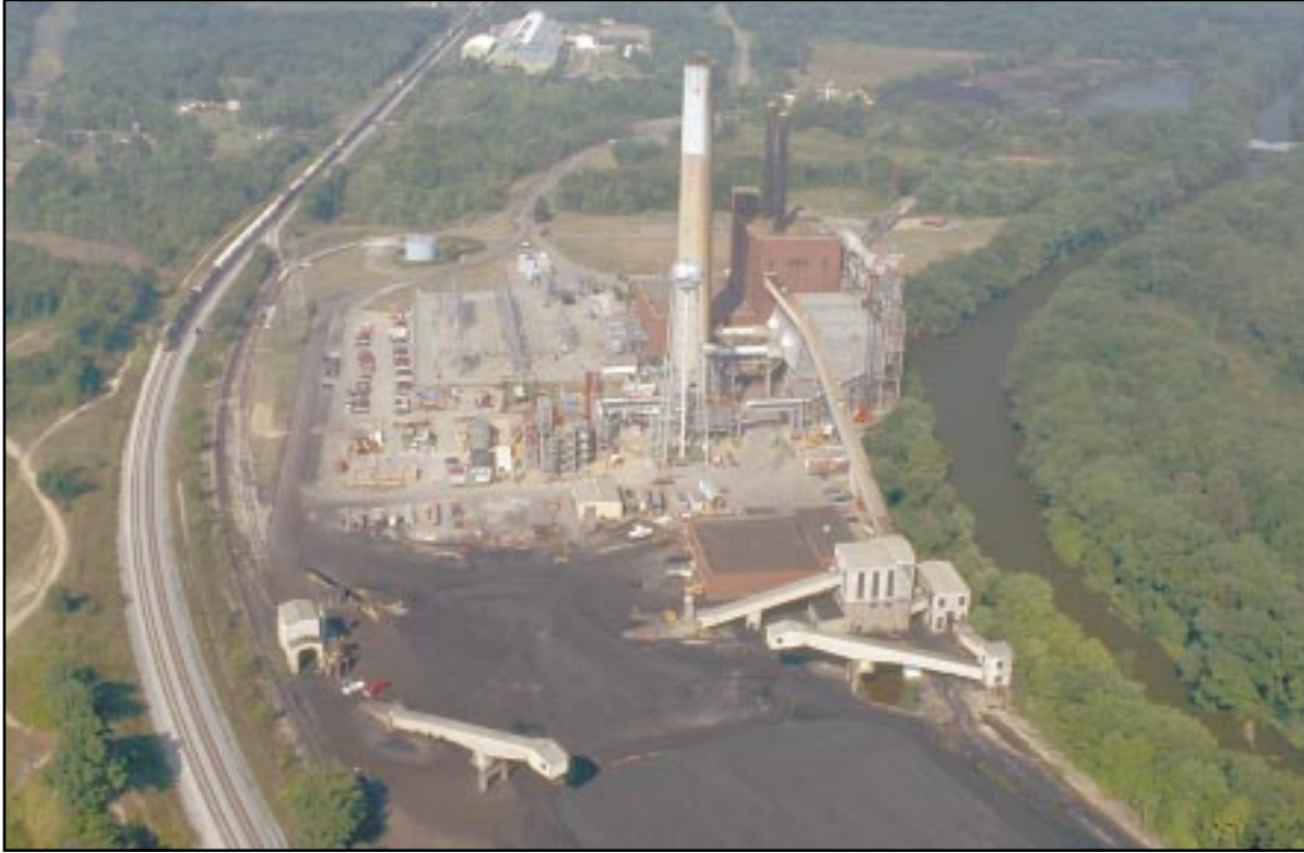
Aerial view of Ohio Edison's Niles Station.
