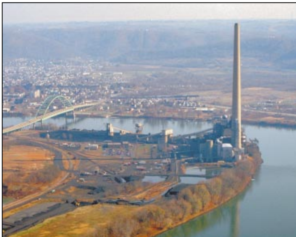
Aerial view of Ohio Edison's R.E. Burger Plant.
