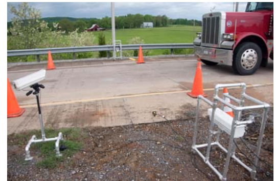
The SIRIS Test System Deployed in the Ramp Leading to the Pit Scale
