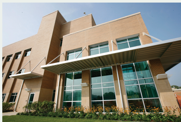
BESC Headquarters. Oak Ridge National Laboratory's new Joint Institute for Biological Sciences facility in Oak Ridge, Tennessee, houses BESC administration and ORNL-based research staff. [Photo courtesy of Oak Ridge National Laboratory]
