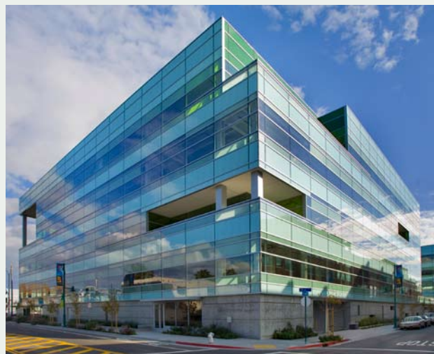
JBEI Research Facility. JBEI researchers are located at a single site in Emeryville, California. [Photo by Roy Kaltschmidt, Berkeley Lab]
