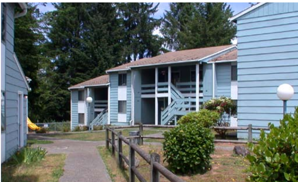
The Oregon Housing and Community Services Department provided financing for Forest Hills, an apartment complex in Reedsport, Oregon, included in the Northwest 12, with 20 units of affordable family housing.
