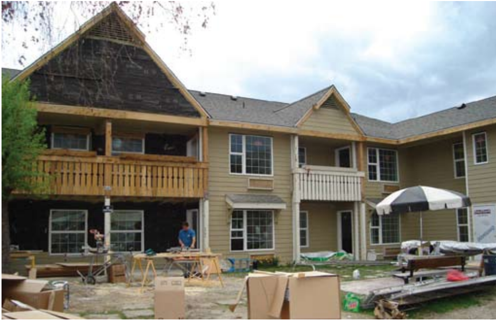
Mercy Housing rehabilitated Cobble Knoll with long-term loans from US Bank.
