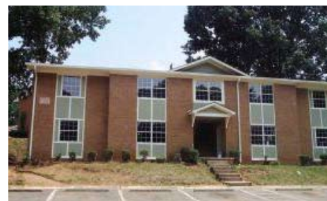
After: The rehabilitated apartments of Flat Shoals.
