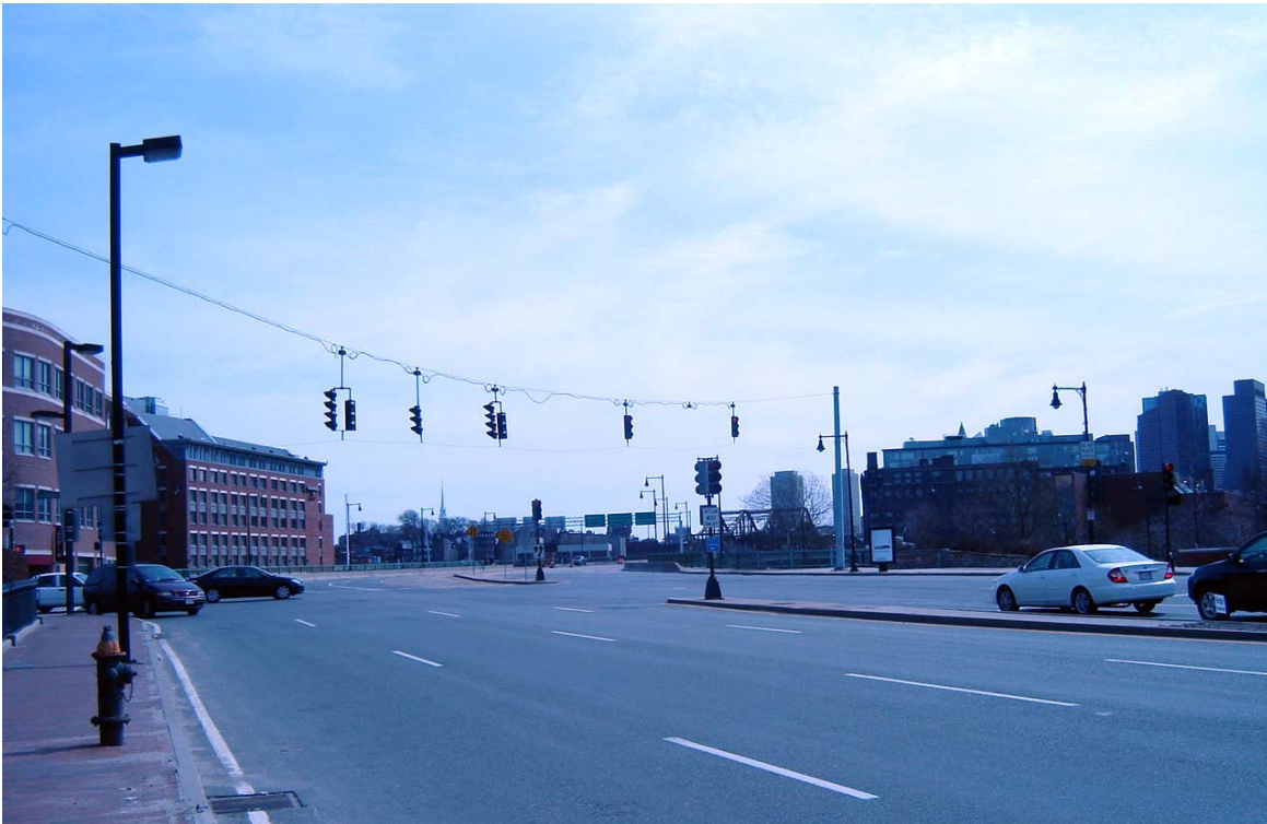
Figure 3-7. Intersection of Route 99 (Rutherford Avenue) and Chelsea Street
