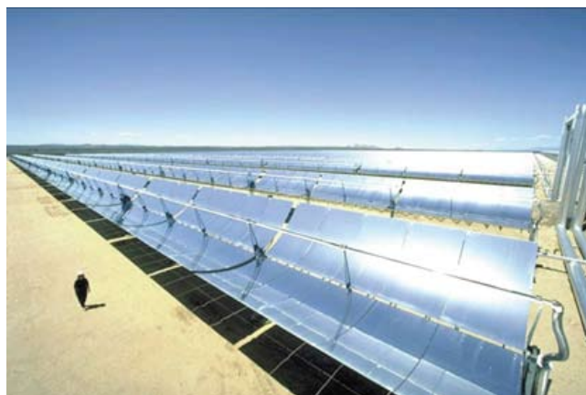
An example of a concentrating solar power U-shaped (parabolic) trough system at Kramer Junction, California.
