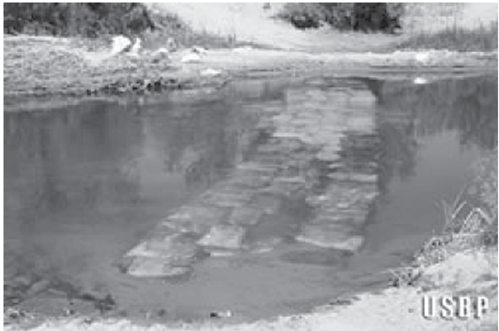
Traffickers constructed this sandbag bridge to transport drugs via vehicles across the U.S.-Mexican border.
