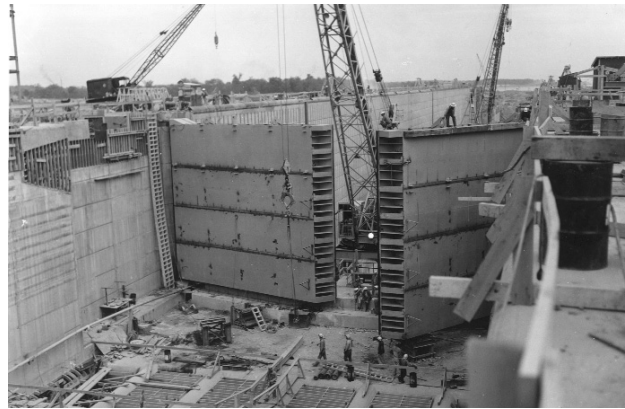
Construction of Snell Lock, August 29, 1957
