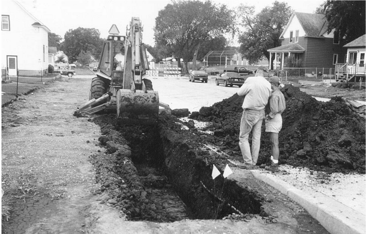
Figure 2.61. Backhoe excavating Block 7, Scattered Village, site 32MO31.
