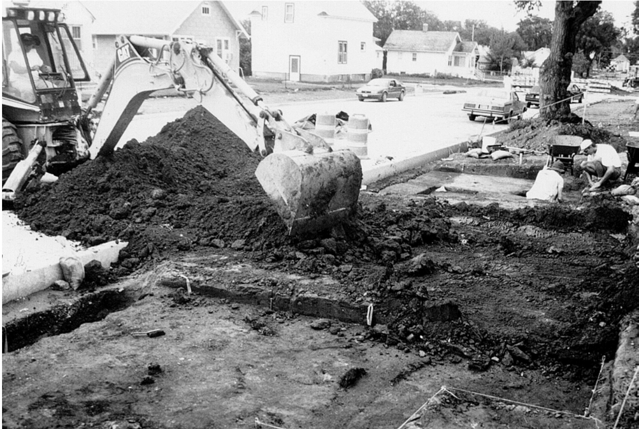
Figure 2.53. Backhoe removing historic overburden, Excavation Block 6, Scattered Village, site 32MO31.
